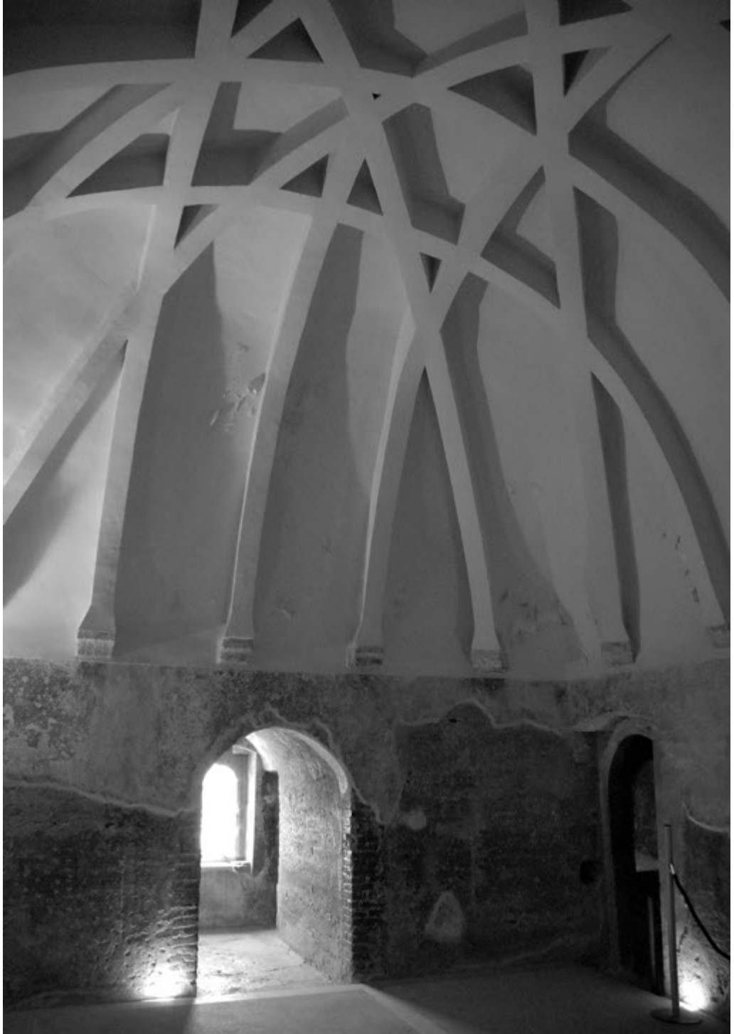
Photo 07. Villena Castle, Spain. Islamic rib vaulting in keep/tower, similar in date and style to one at Biar castle nearby
