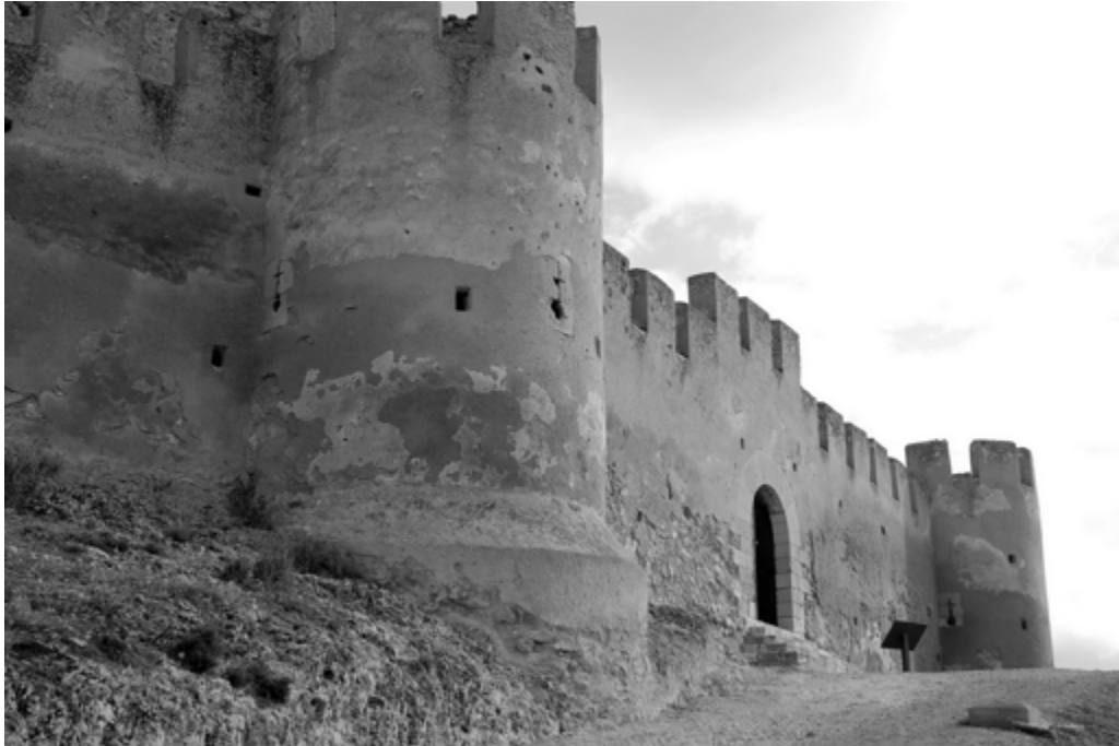
Photo 15. Castillo de Biar, Spain. Outer curtain, gateway and corner towers - post-Islamic period replacements.
