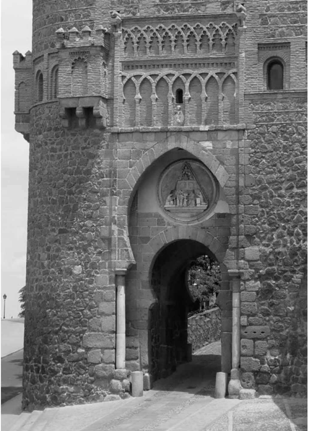
Photo 11. Toledo, Spain. Puerta del Sol. Gateway into town – 13 th C.
