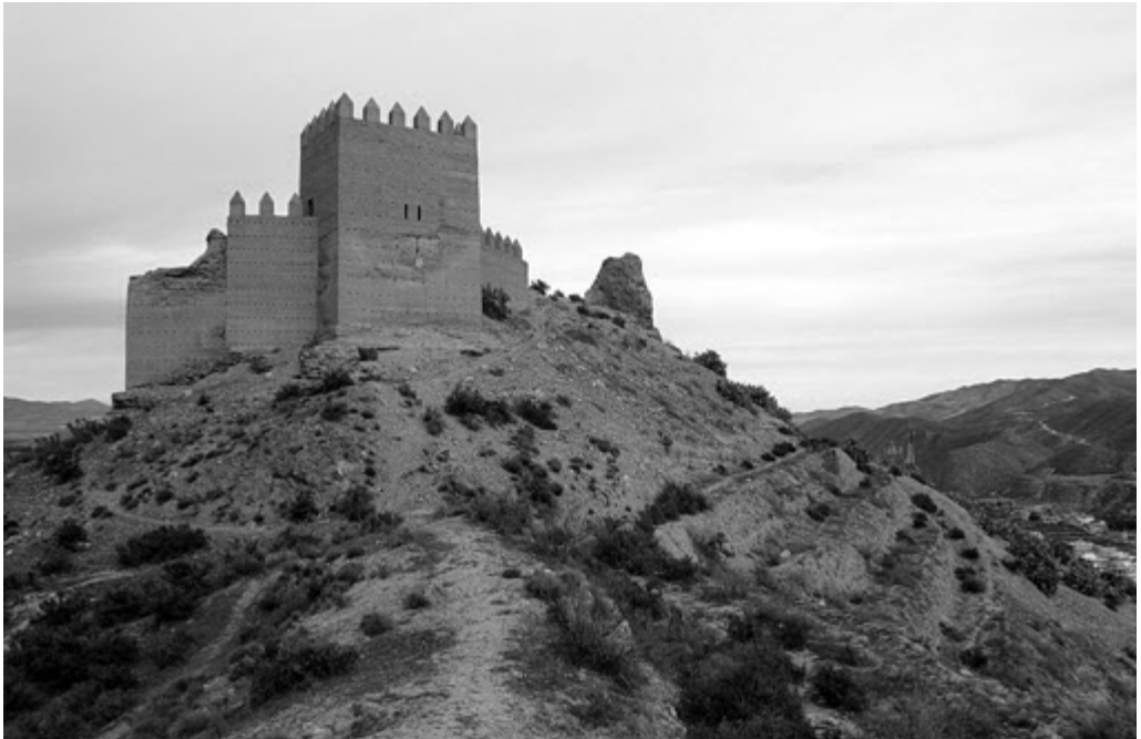
Photo 01. Tabernas Castle, SE Spain nr. Almería. Tapial construction on hilltop site.
