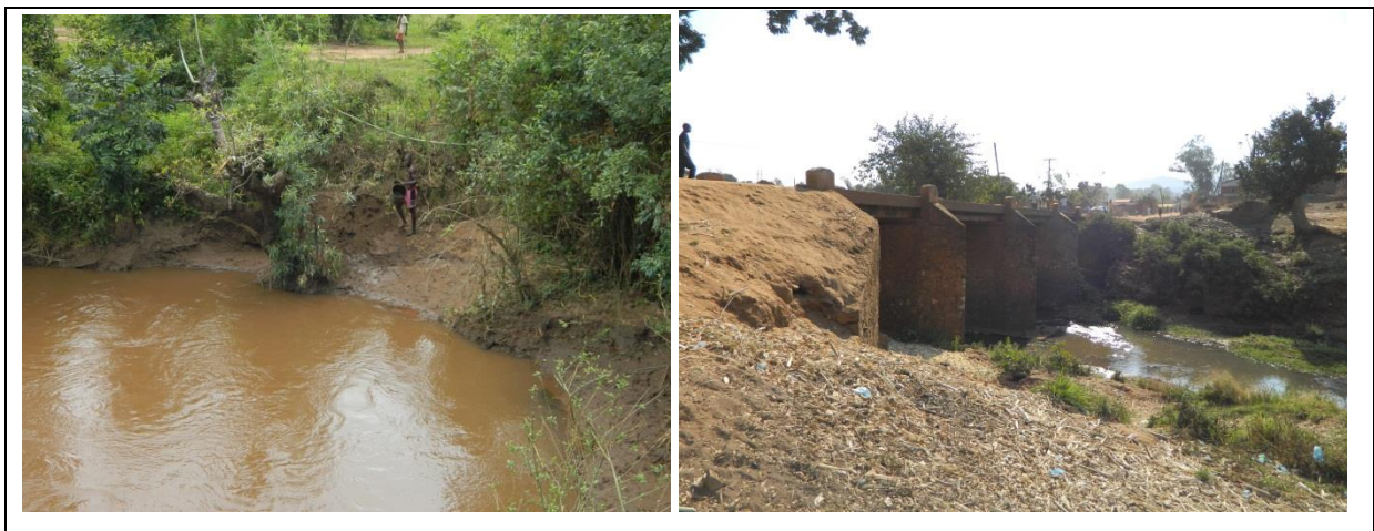
Figure 28: Sand mining along Likangala River and solid waste disposal at Mpondabwino
