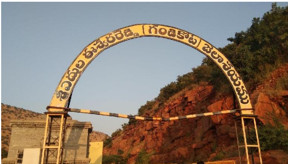
View towards Entrance of Gandikota Dam
