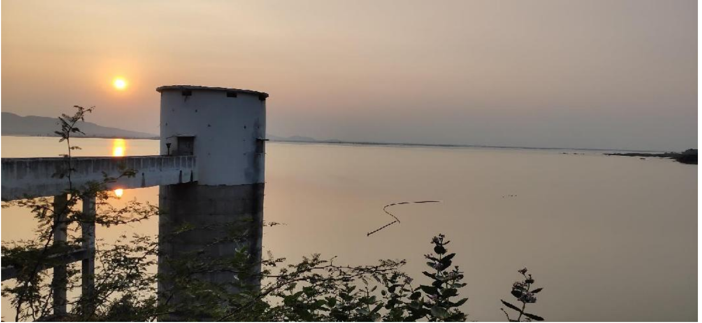
Existing Pump Room – Gandikota Dam – Lower Reservoir
