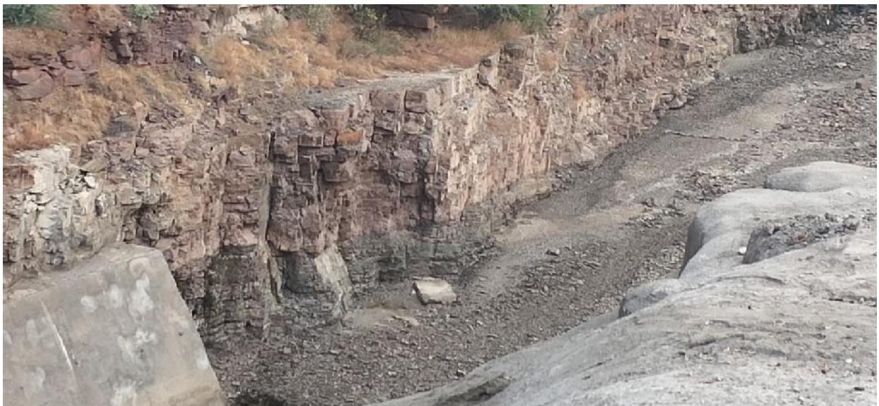
Existing Tunnel from Srisailam/ OWK Reservoir near to Proposed Upper Reservoir
