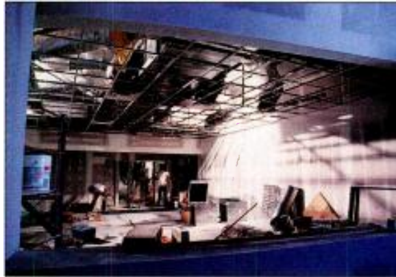
The CNN/SI facility under construction
