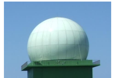
Fixed warning and control radar (FPS-7)
