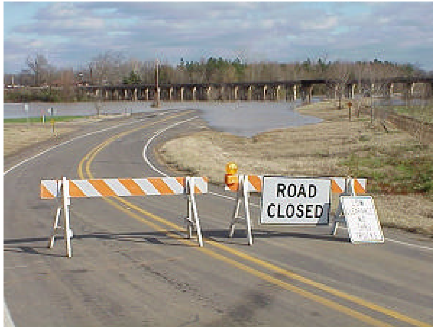
Arkansas Highway 7 was under water at a railroad underpass in Arkadelphia (Clark County) on 12/17/2001.
