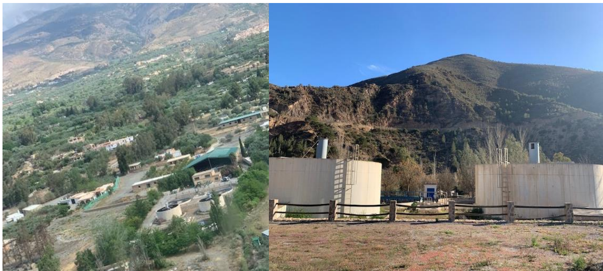
Figure 6. Wastewater treatment plant in Órgiva, Granada.
