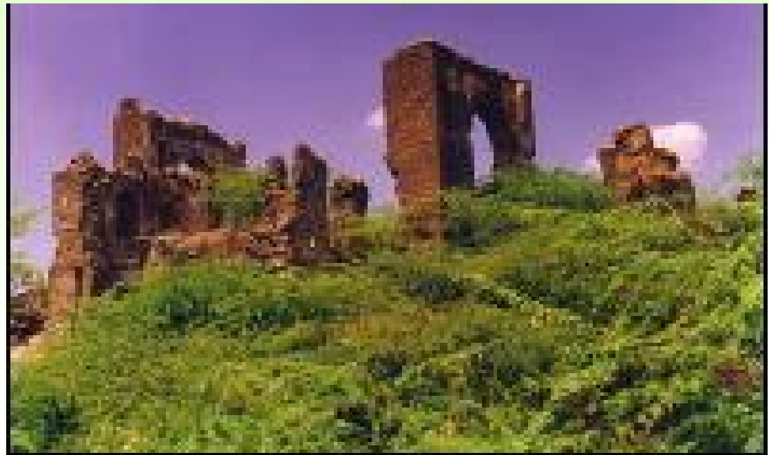
Ruined Citadel Walls of Bijapur
