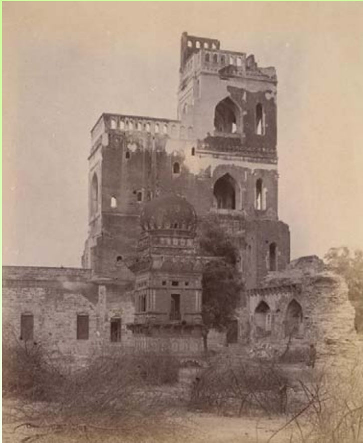
View from the North Side of the Sat Manzili: (Henry Cousens, 1880s)
