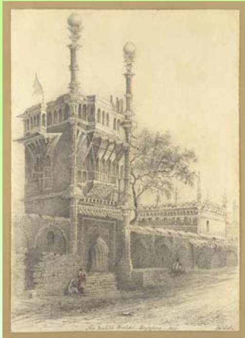
Another View: Main Façade (Henry, Hardy Cole, 1880)
