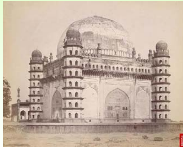
Gol Gumbaz: General View from South East, (Cousens, 1880)
