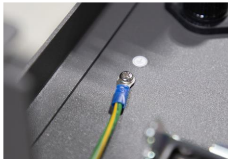
Figure 22: Securing the ground wire with control box
