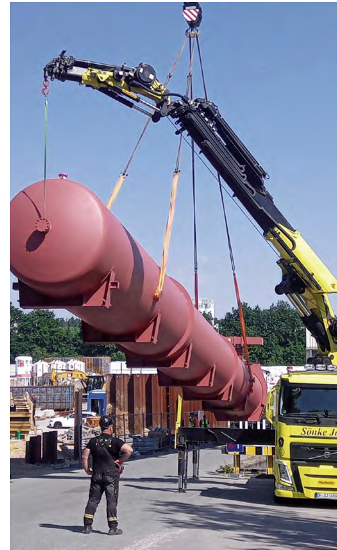
Crane unloading new autoclave in Wittenborn, Germany
