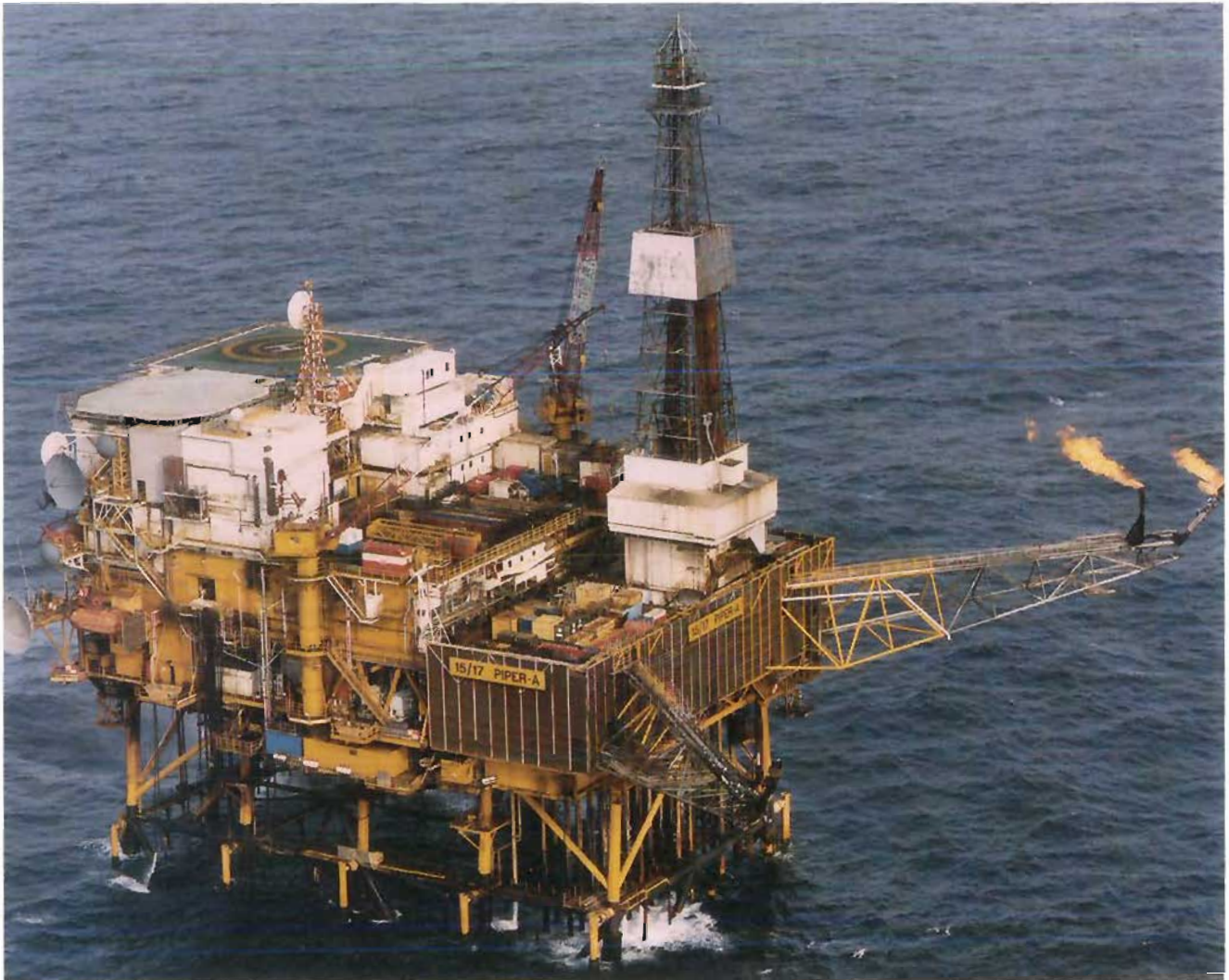
Plate 5 The Piper Alpha platform: west face and pipe deck.
