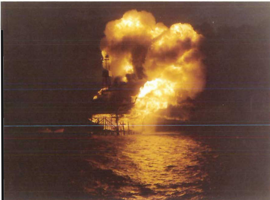
Plate 19(b) The fires on Piper just after rupture of the Tartan riser: photograph taken by Mr Gibson from the Lowland Cavalier at a time estimated as 22.20–22.22 hours.
