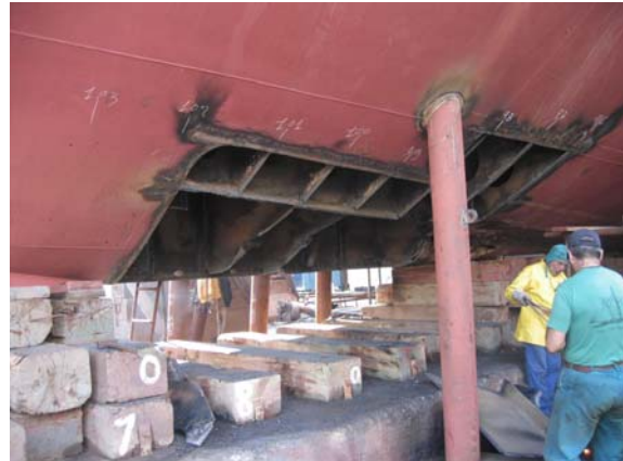
Figure SMO 6 Hull repairs to NRV Alliance.
