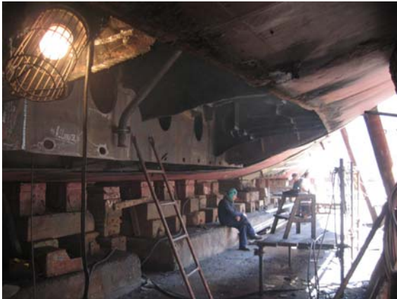
Figure SMO 5 Hull repairs to NRV Alliance.
