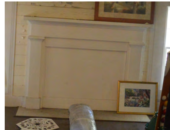
Figure 47. (Photo 35) Smaller and simpler fireplace surround and mantel in Room 203.
