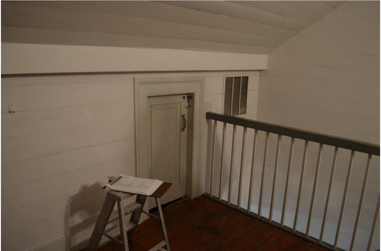
Figure 75. (Photo 62) Room 201, Southeast corner with door to 204
