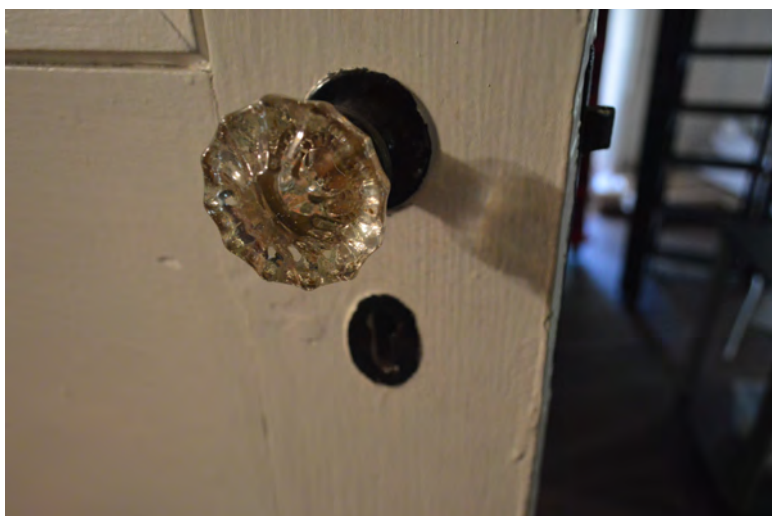
Figure 80. (Photo 67) Glass doorknob entering room 203 from 201
