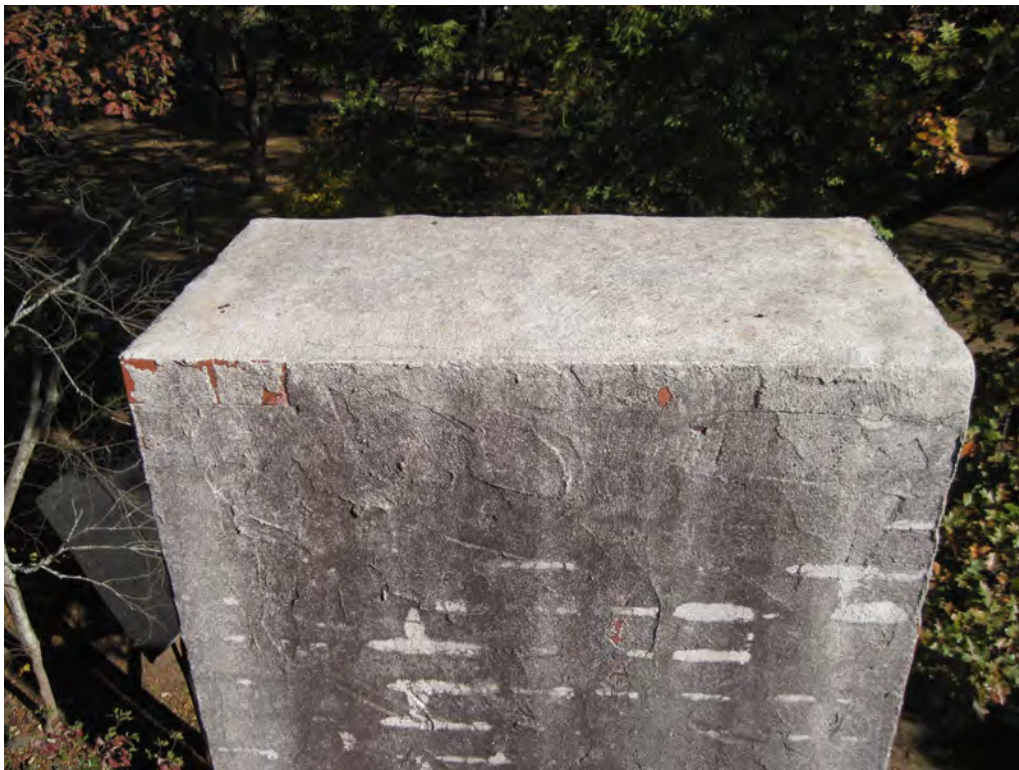
Figure 18. (Photo 12) View of concrete cap on northwest chimney
