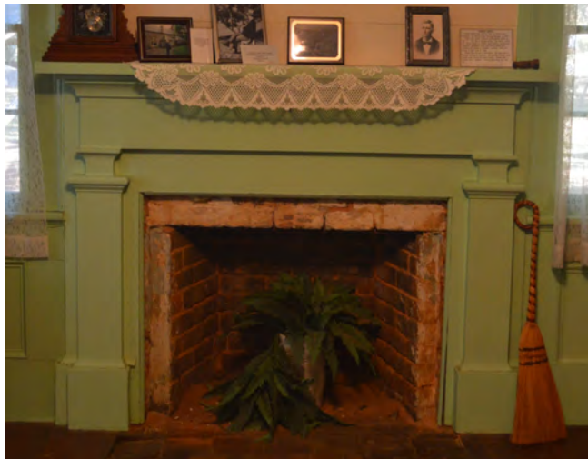
Figure 44. (Photo 32) Fireplace surround and mantel in the Room 103 displaying the brick firebox and hearth
