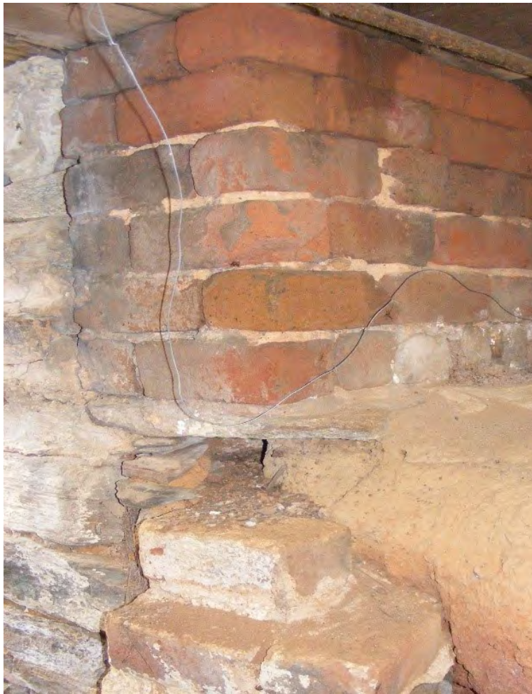
Figure 19. (Photo 13) View of foundation
