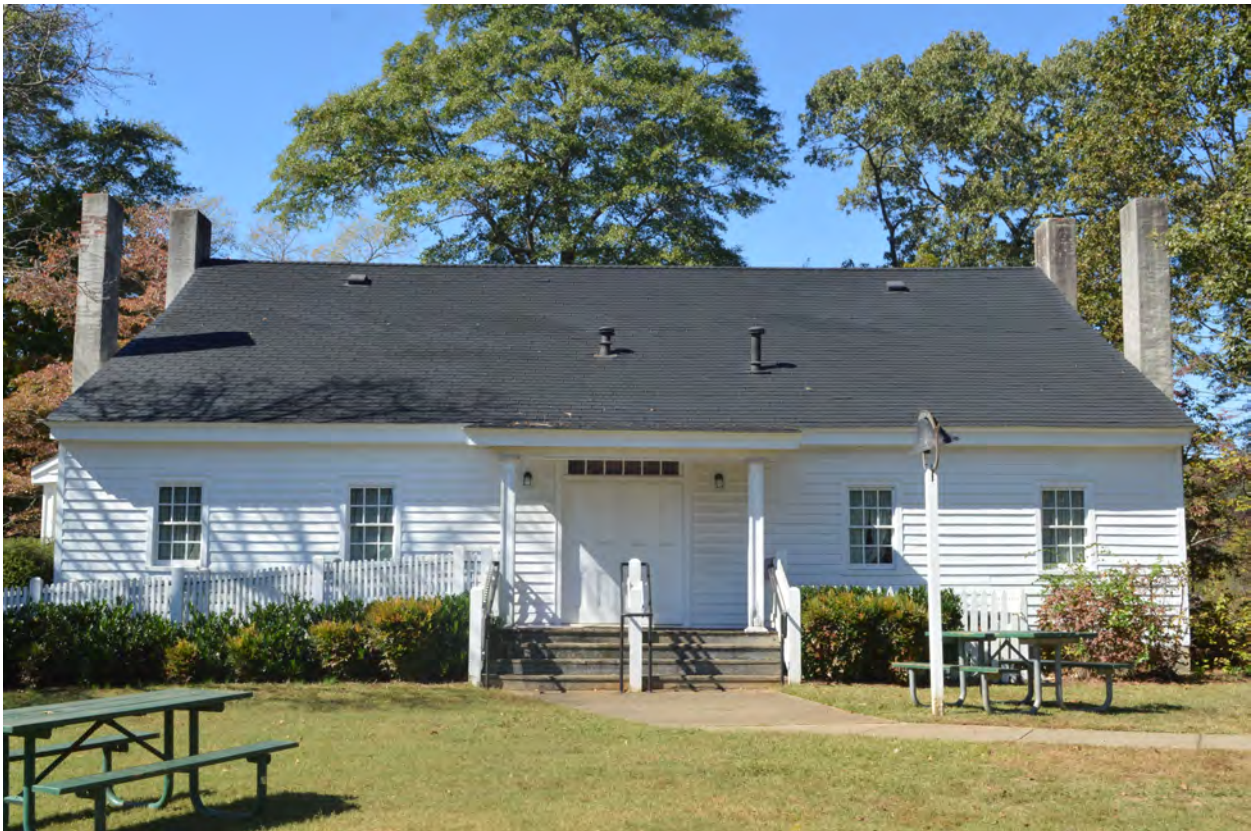
Figure 24. (Photo 16) View of east façade
