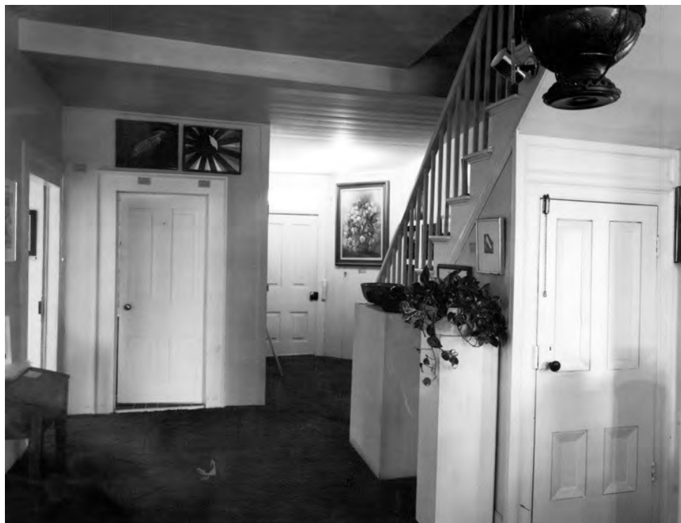
Figure 38. Room 101 facing east showing where bathroom was once installed but later removed, photo by James R. Lockhart in 1986
