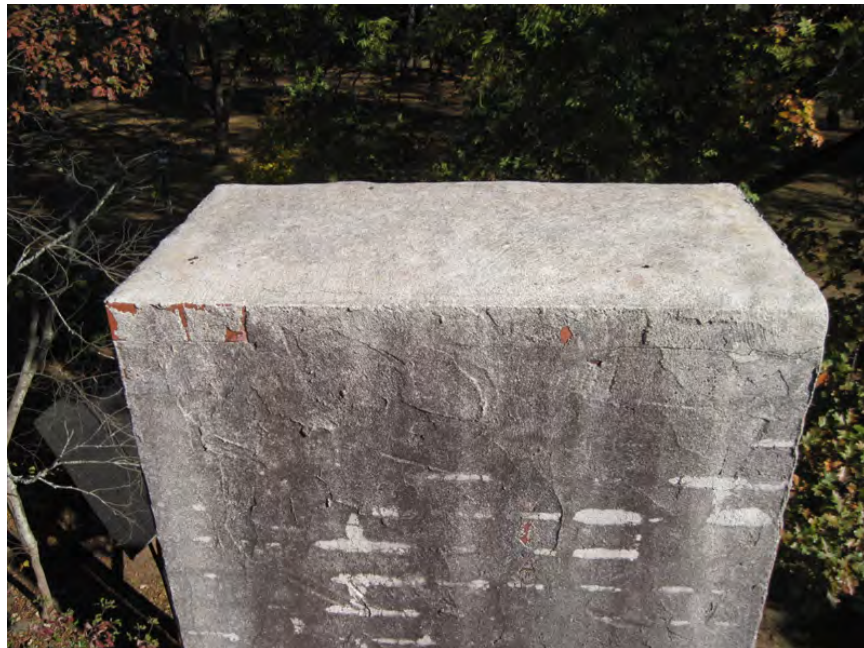
Figure 30. (Photo 20) View of concrete cap on northwest chimney
