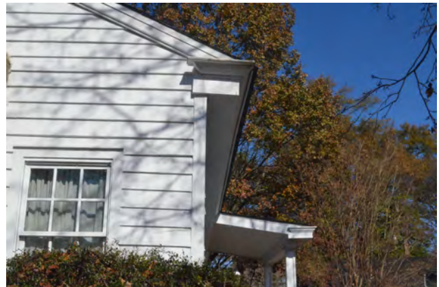
Figure 29. (Photo 19) View of Cornice Return
