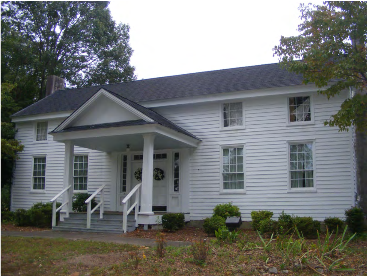
Figure 20. (Photo 14) View of west façade
