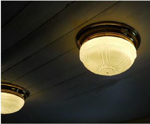
Figure 42. (Photo 30) Light fixtures in room 104
