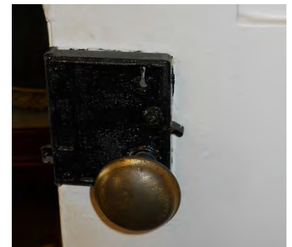
Figure 40. (Photo 28) Metal rim lock and doorknob, D7
