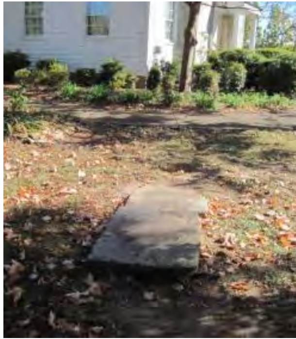
Figure 14. (Photo 9) View of cracked hearthstone, looking southeast
