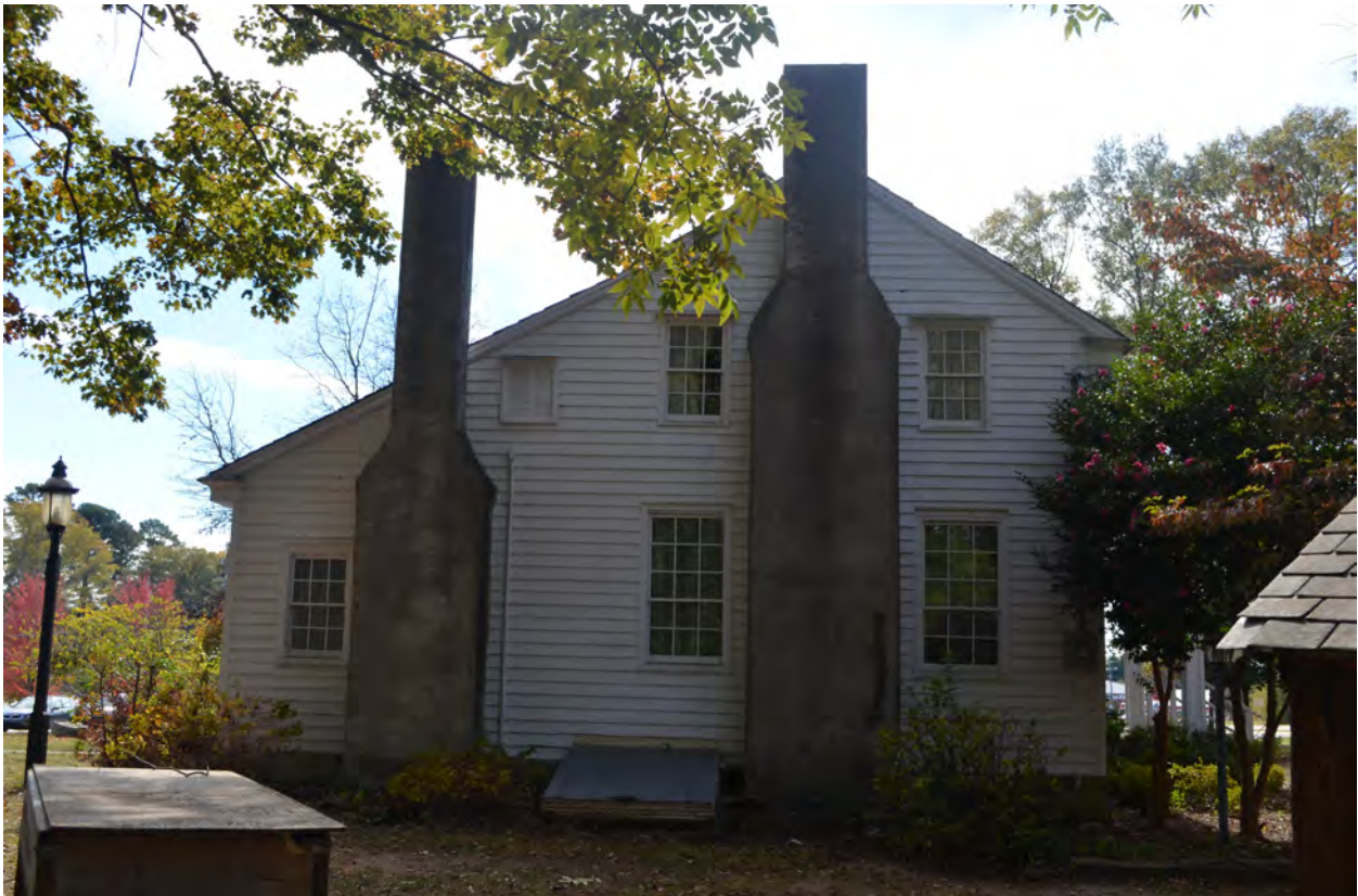
Figure 26. (Photo 17) View of north façade
