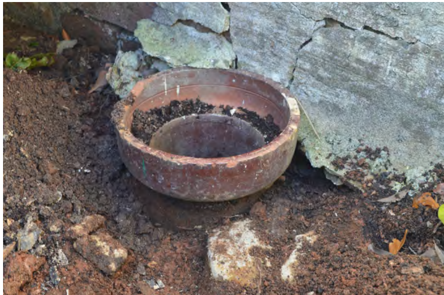
Figure 116. (Photo 99) Terracotta drainage hole on east facade
