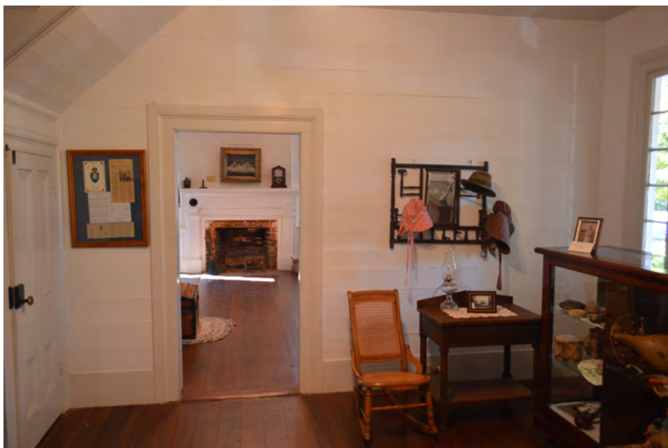
Figure 58. (Photo 46) The wide beaded baseboard in Room 101.
