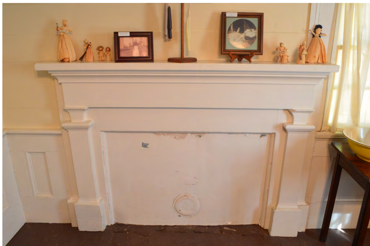
Figure 67. (Photo 55) Room 105, pilaster mantle with sealed opening
