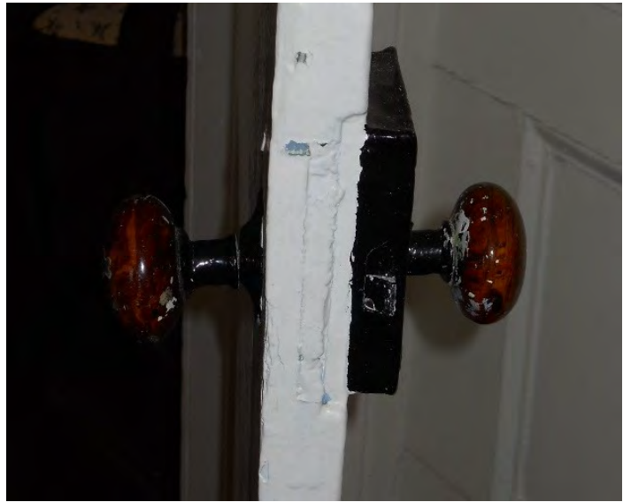
Figure 37 (Photo 26) The mortise and tenon construction method is visible on the door's edge, as seen in the photo to right.
