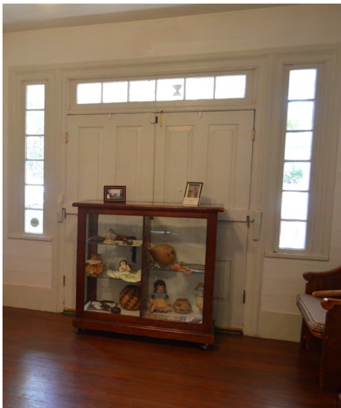
Figure 55. (photo 43) Front entry doors on west wall, room 101
