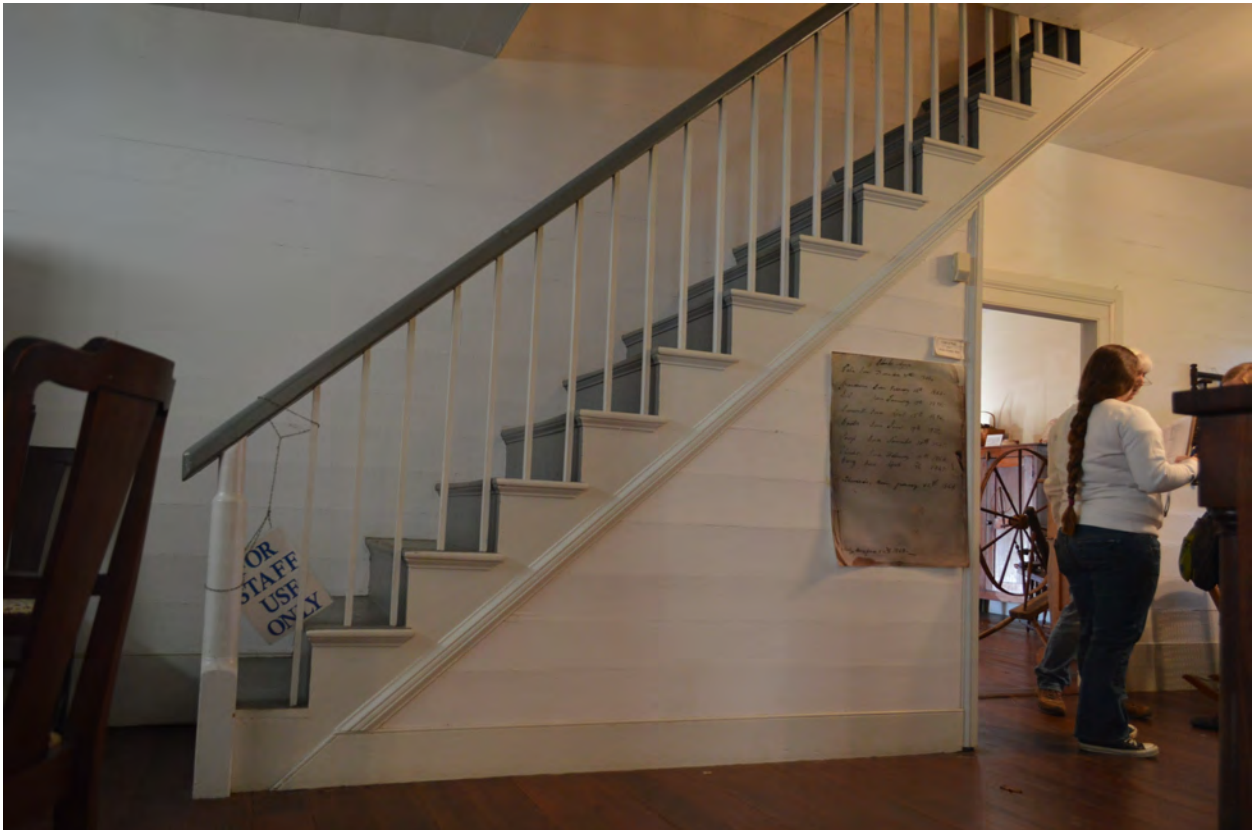
Figure 73. (Photo 60) Turned detail on newel post
