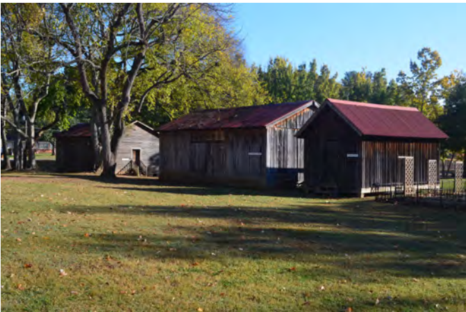
Figure 12. (Photo 7) View of west facades of outbuildings from Main House; from left to right: sweet potato house, blacksmith shop, corn crib and garden
