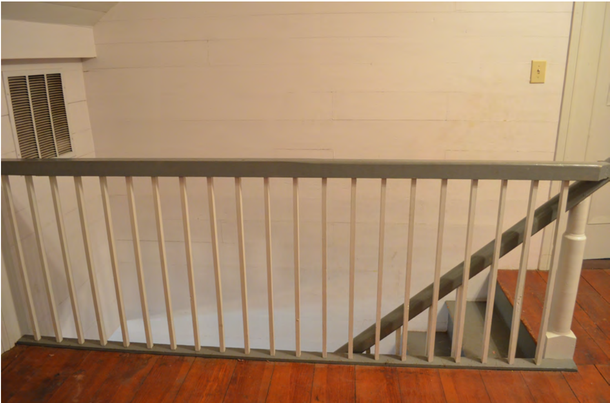
Figure 76. (Photo 63) Room 201, staircase along south wall showing simple square balustrades and turned detail on newel post
