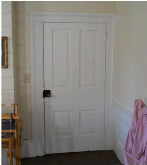
Figure 36 (Photo 25) Room 105 door viewed from inside the room.
