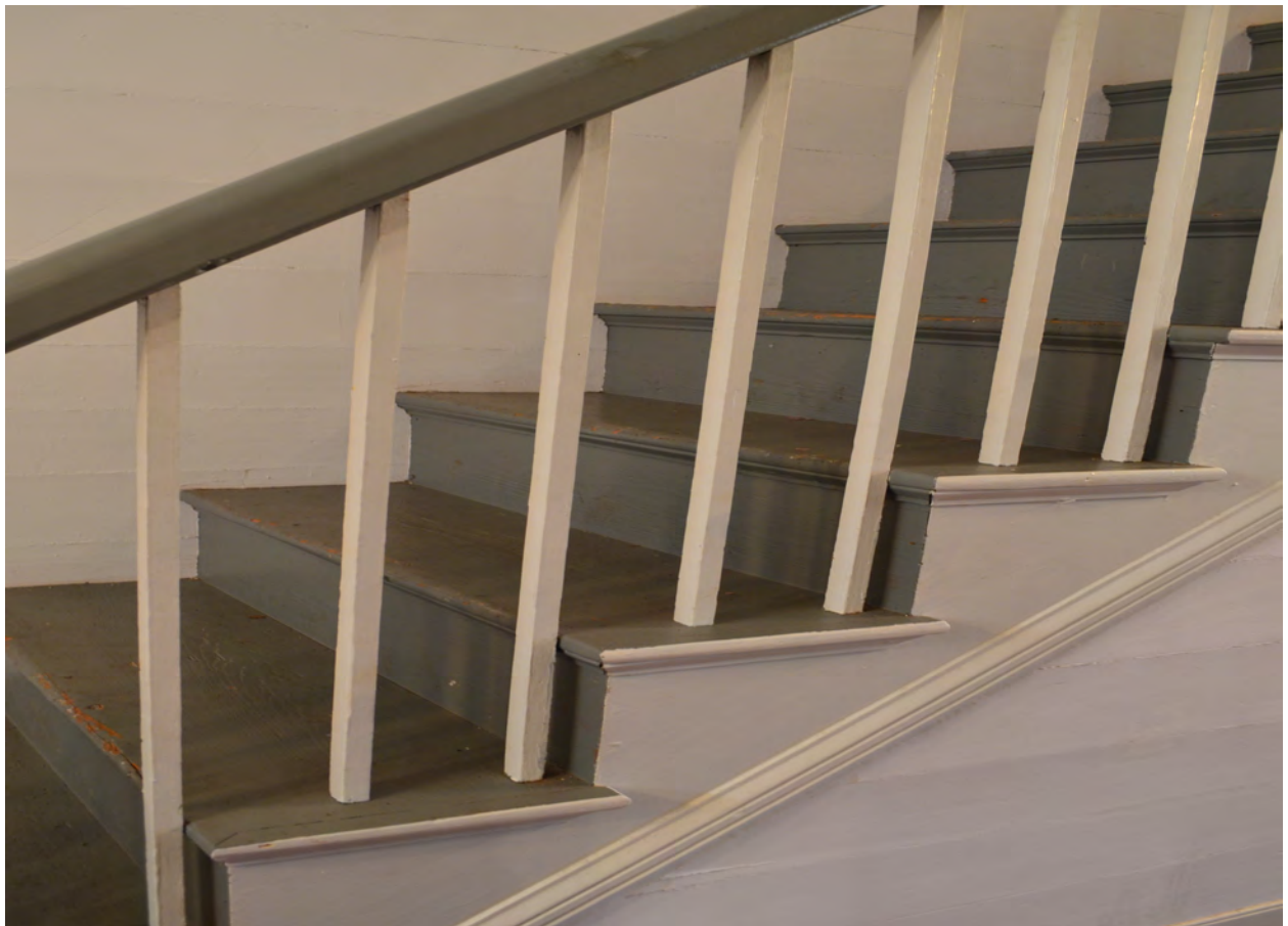
Figure 71. (Photo 58) Simple square balusters
