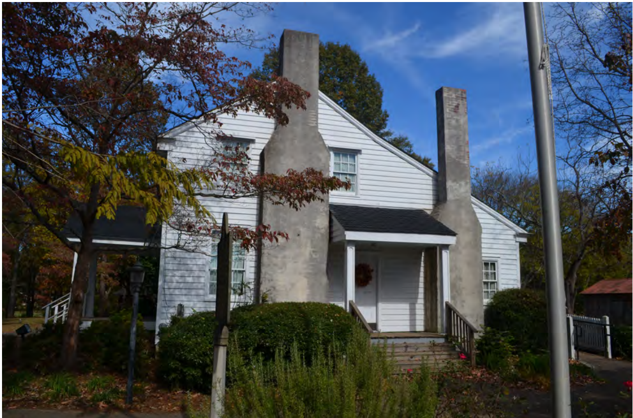
Figure 22. (Photo 15) View of south façade
