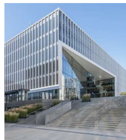
Fig. 64 Danske Bank offices (2016).
