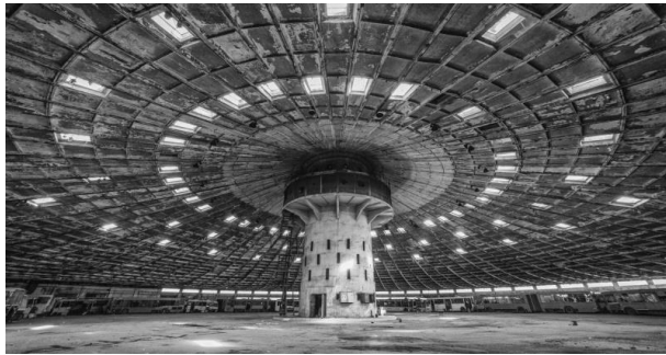
Fig. 27. Roof of bus fleet
