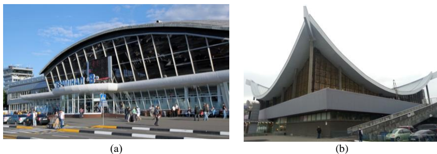
Fig. 11. Shell roofs: (a) - airport terminal in Boryspil, (b) - furniture house in Kyiv
