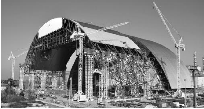
Fig. 28. Installation of confinement structures
