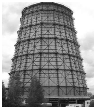
Fig. 4. Cyclically symmetric frame of a cooling tower
