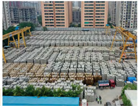
Segment Casting for Tunnel
