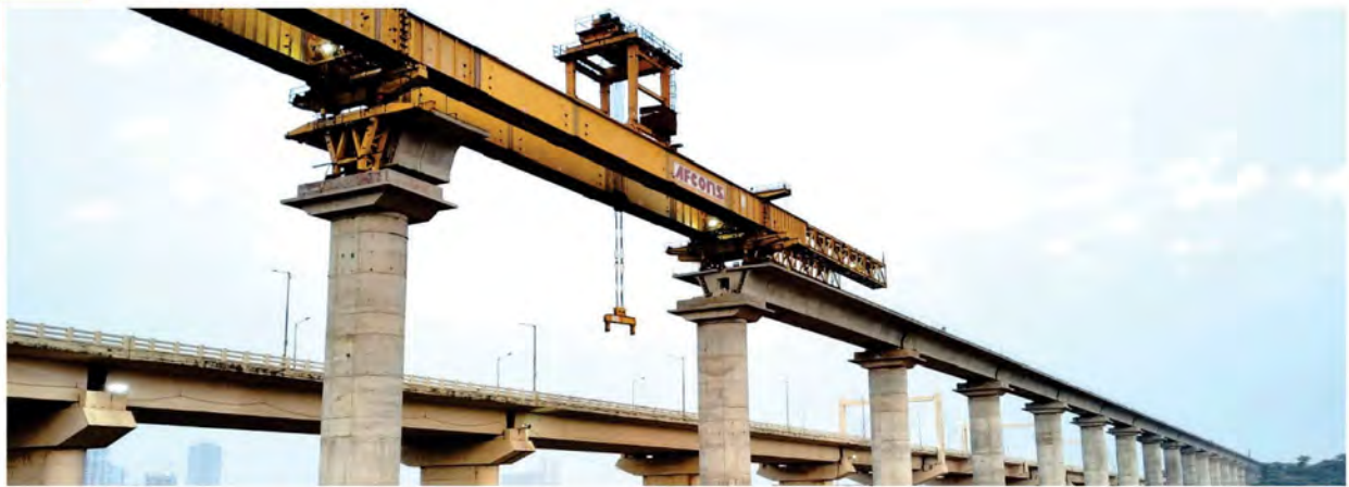
Sabarmati River Bridge
