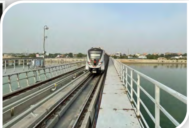
Trainset Testing on Mainline
