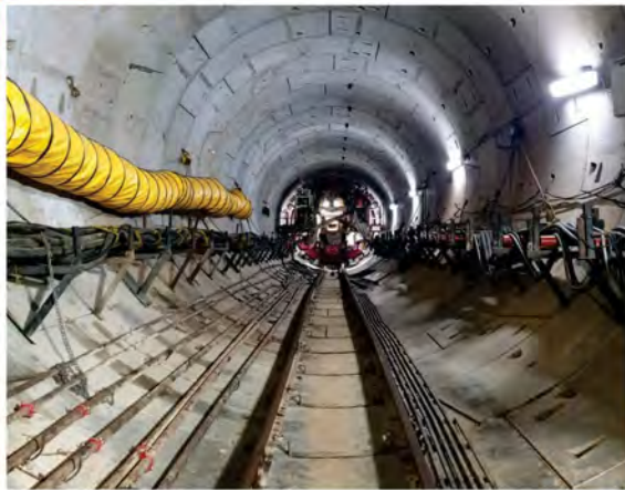
Tunnel Works at Kapodara
