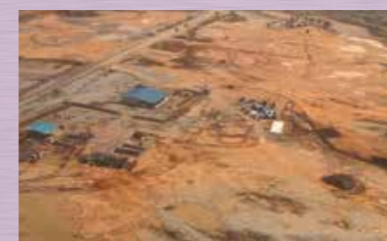
Construction of Samalaju Industrial Park begins in 2009
