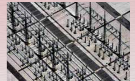
In June 2011, Sarawak Energy Bhd and Sarawak Hidro Sdn Bhd signed the 30-year Power Purchase Agreement (PPA) for the full output of the Bakun hydroelectric facilities
