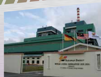
Mukah coal-fired power plant starts operations in April 2009
