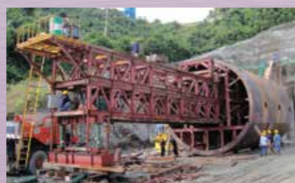
Construction of Murum Dam begins
