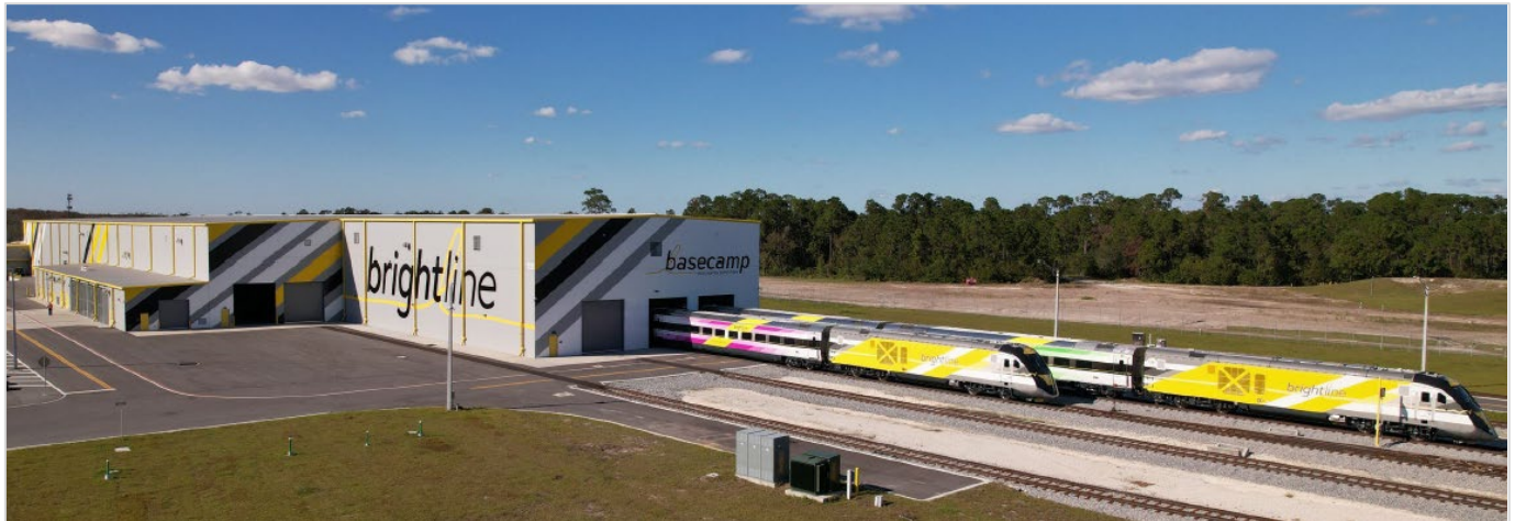
Aerial view of Vehicle Maintenance Facility, December 20, 2022
