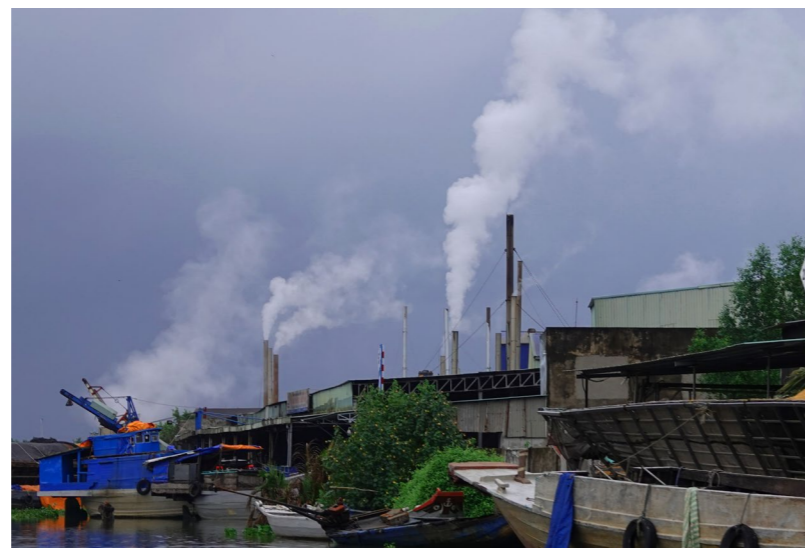
FMFO plant at Kien Giang
