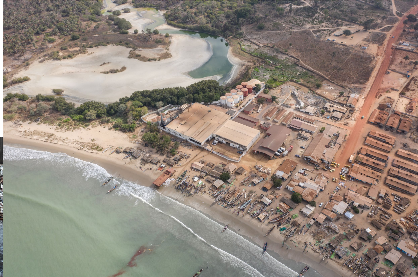
Aerial view of the Golden Lead plant at Gunjur
