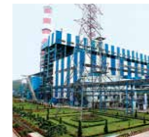
CAPTIVE POWER PLANT JINDAL STEEL & POWER LTD. Dongamahua, Chhattisgarh, India
