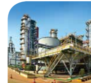
INTEGRATED STEEL PLANT JINDAL STEEL & POWER LTD. Angul, Odisha, India
