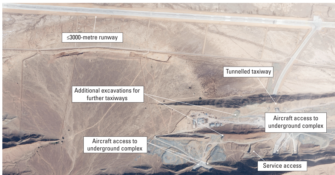
Figure 7: Oqhab 44 air base (under construction) (28.04558, 55.52038), 21 February 2023
