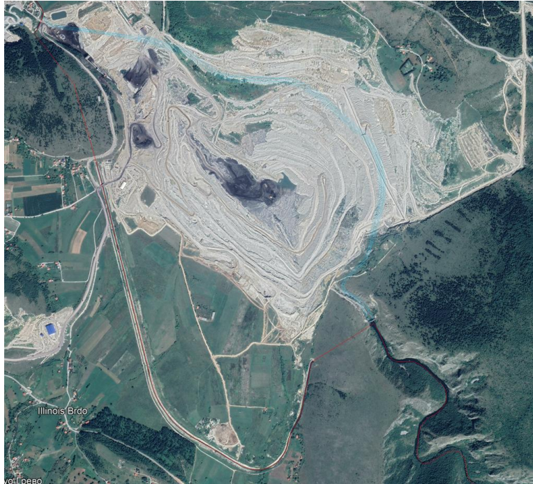
Figure 2 State of works at the Potrlica open pit (Google Earth satellite image)
