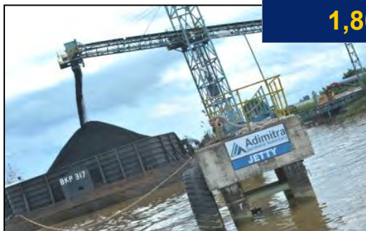
Barge Loading Jetty
