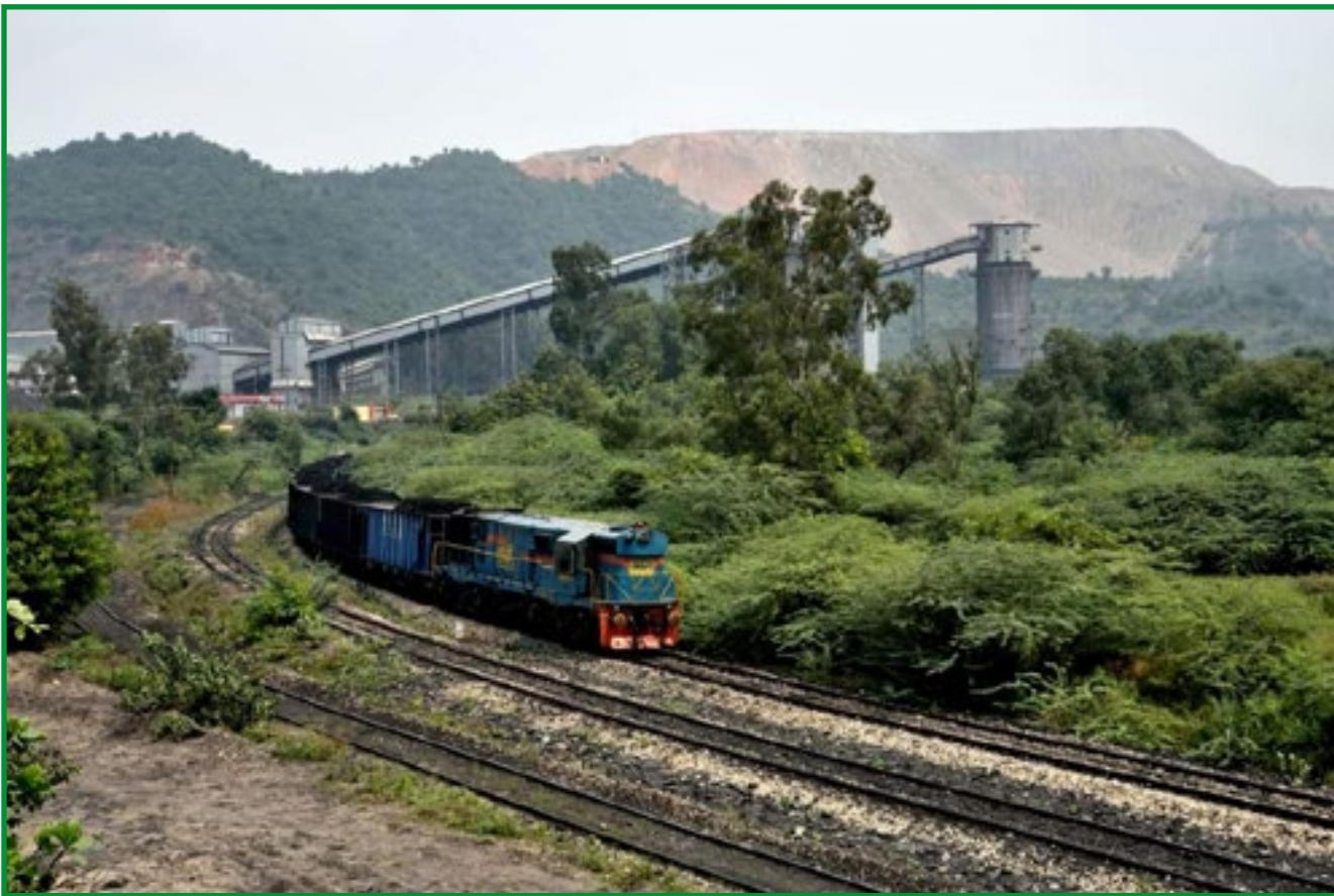
Coal Transportation through CHP-SILO loading system
