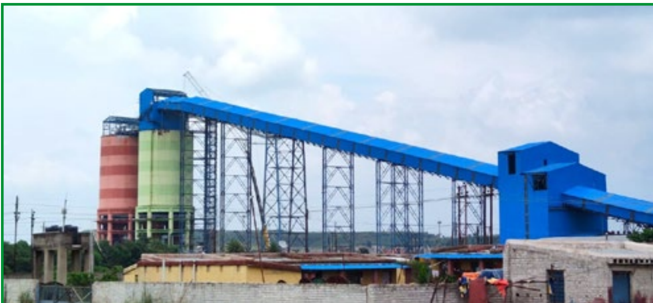
CHP & SILO at Sonepur Bazari Area of ECL
