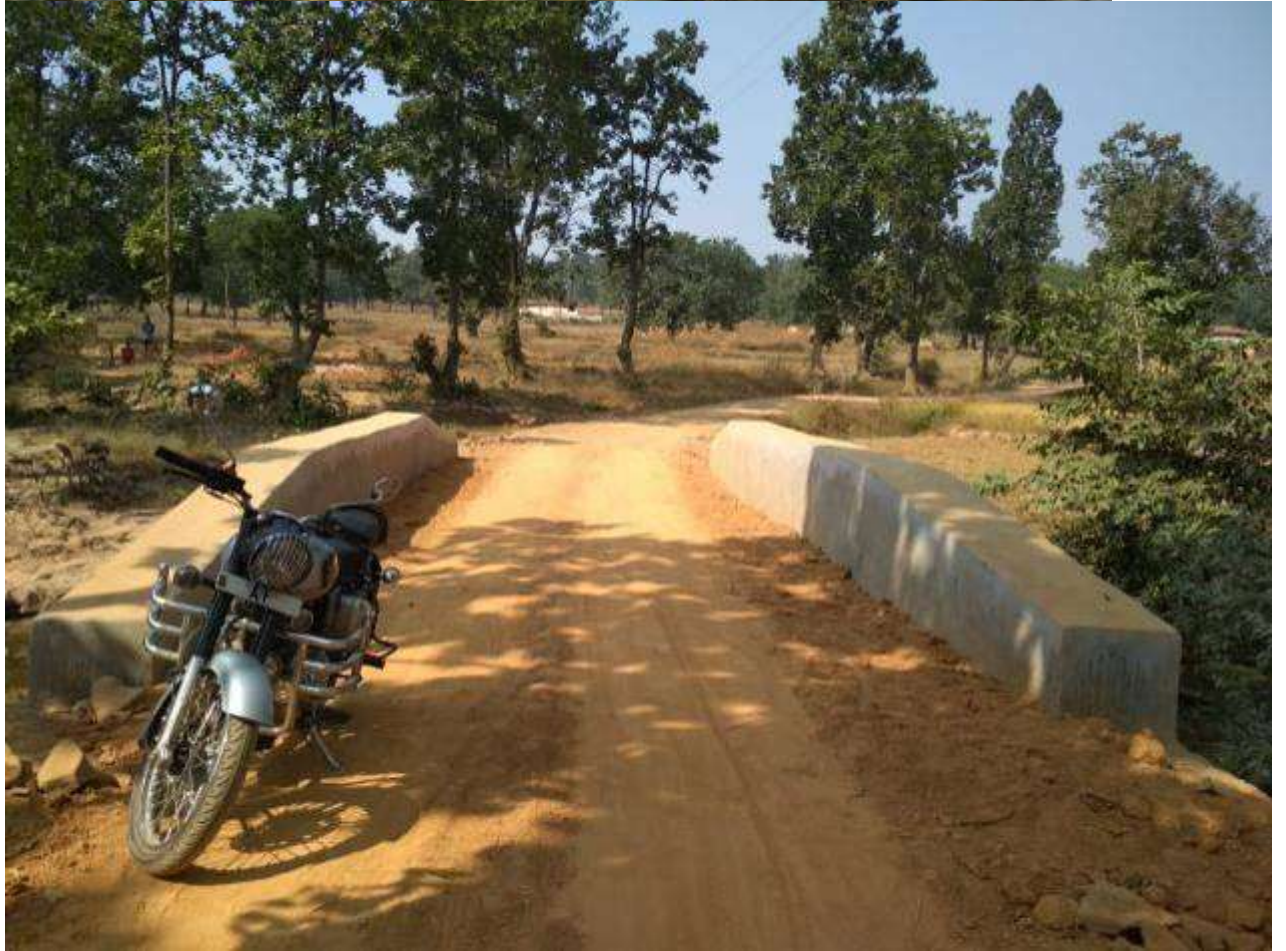
Construction of road and bridge near Purnadih village
