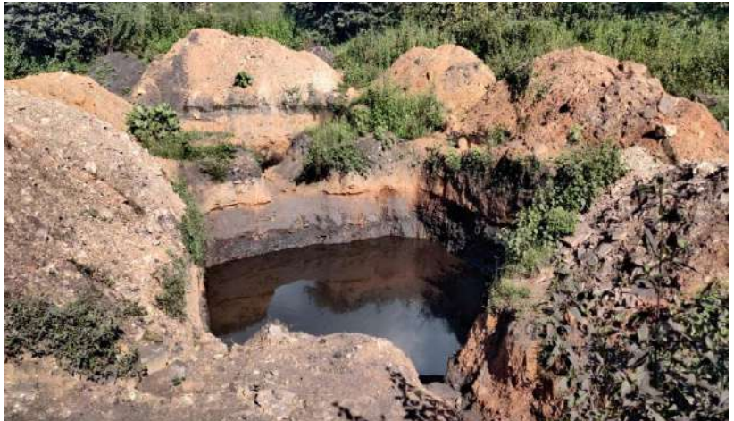
Eight sedimentation ponds constructed all over the projects to arrest silt.
