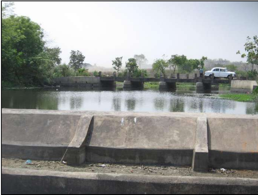
Figure No-2: Check Dams / Nala bunds.
