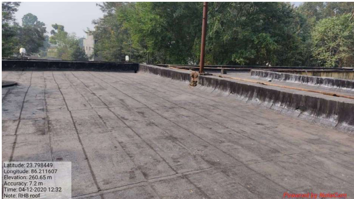
Proposed Rain Water Harvesting Site Regional Hospital Baghmara, Cluster-I, Barora Area
