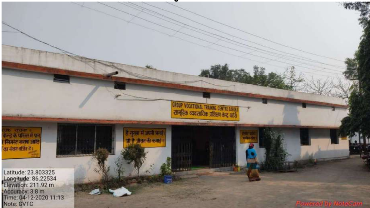
Proposed Rain Water Harvesting Site GVTC, Cluster-I, Barora Area
