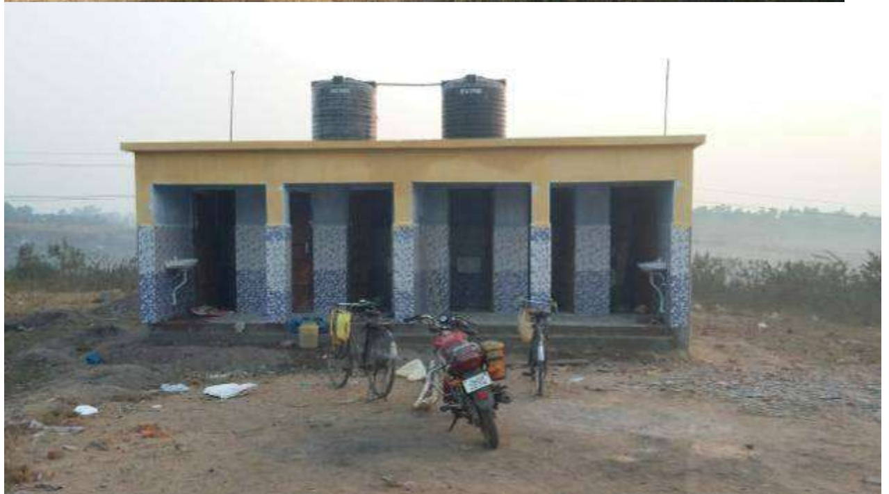
Construction of toilets
