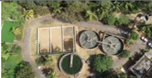
STP (1.5 MLD) Rudrampur Colony, Kothagudem
