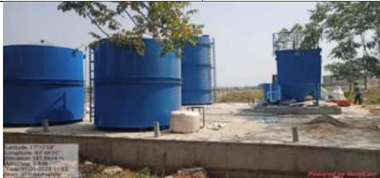
200KLD STP under construction at Sathupalli
