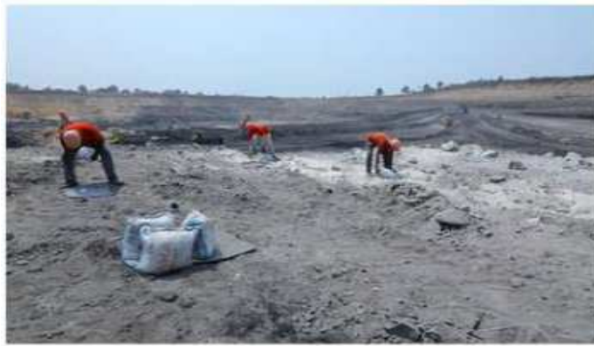
Muffled blasting technic (controlled blasting)
