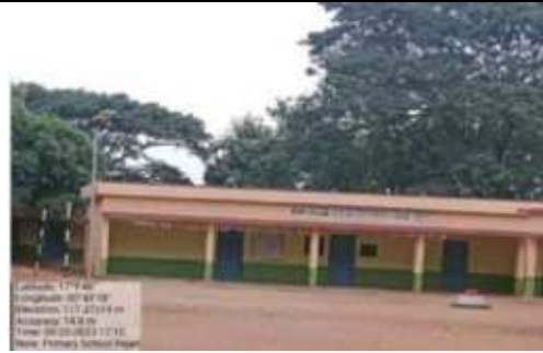
Class rooms at Rererla Village ZPHS
