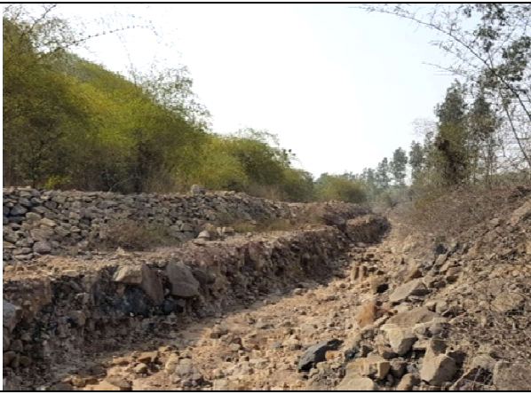
Toe walls and Garland Drains along internal Dump of JVR OC-I Exp
