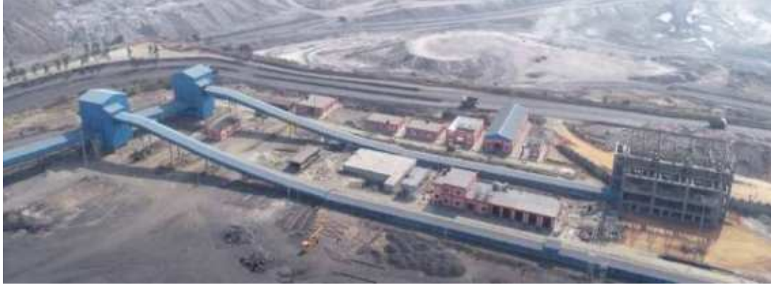
New CHP along with closed belt conveying system
