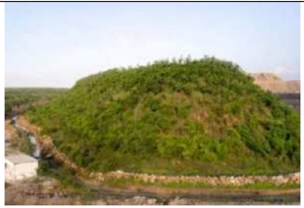
Toe walls and Garland Drains along internal Dump of JVR OC-I Exp
