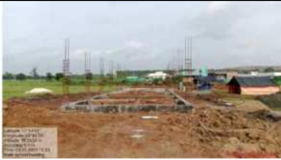
Construction of new school buldin in Jagandapuram
