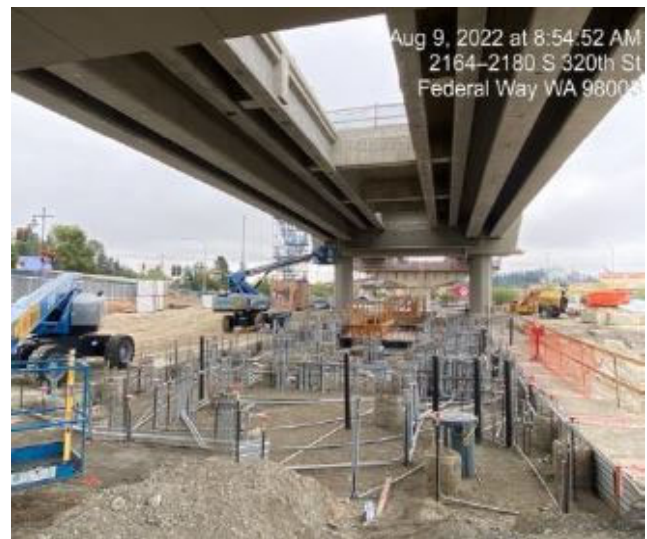
WA3.8 FWTC Soffit Steel Install
