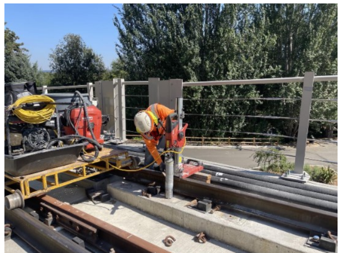
Crews Coring Plinths for Fastener Insert Re-installation
