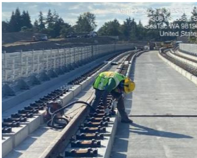
WA1.1 Direct Fixation Track Grinding
