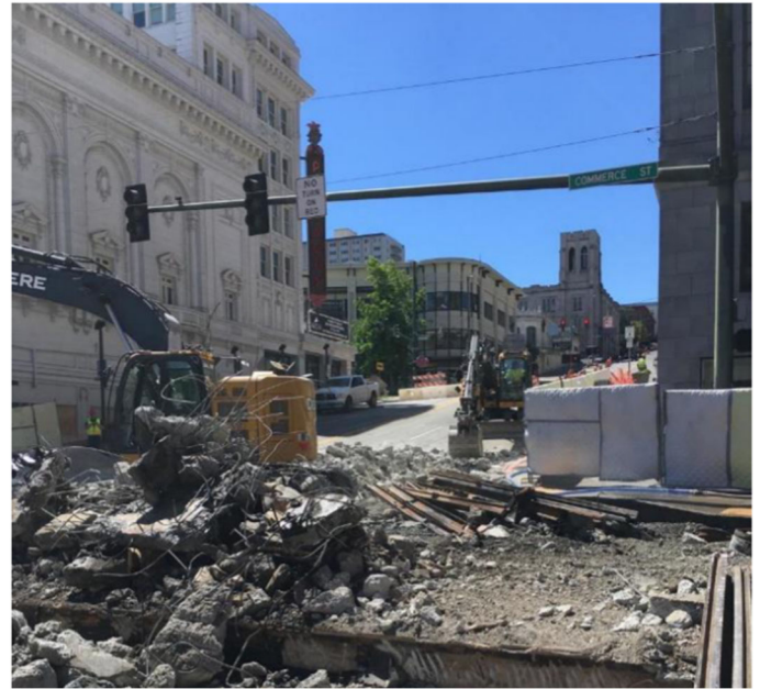
Removing switch at 9th and Commerce
