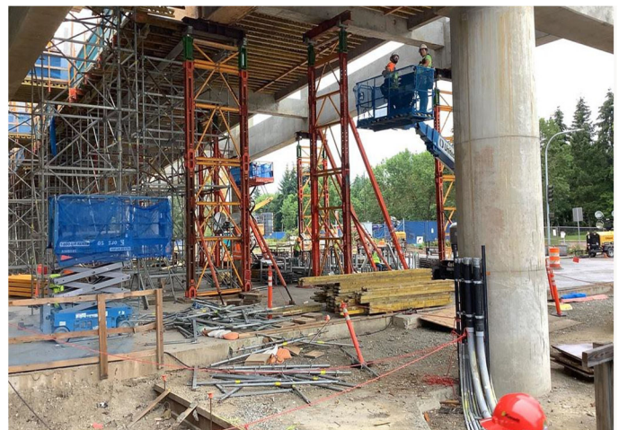
Shoring Removal at RTS Garage Rebuild.
