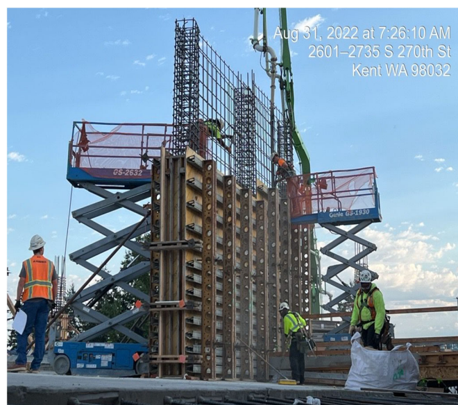
WA 2.4 SL Garage Concrete Placement for Shear Wall on PJ
