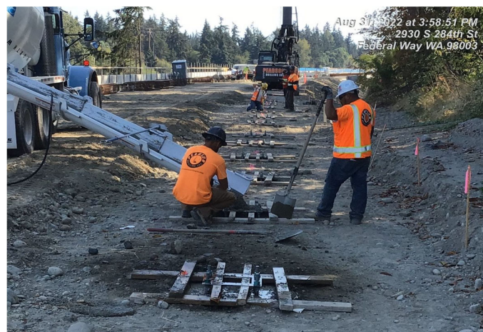
WA 3.3 Pearson Place Concrete at 1264 Drill Shafts - S.JPG
