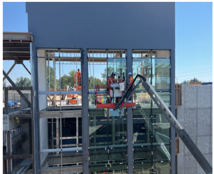
Lynnwood Station Elevator Glass Installation
