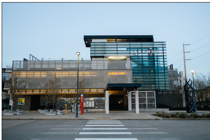
Lakewood Station Garage
