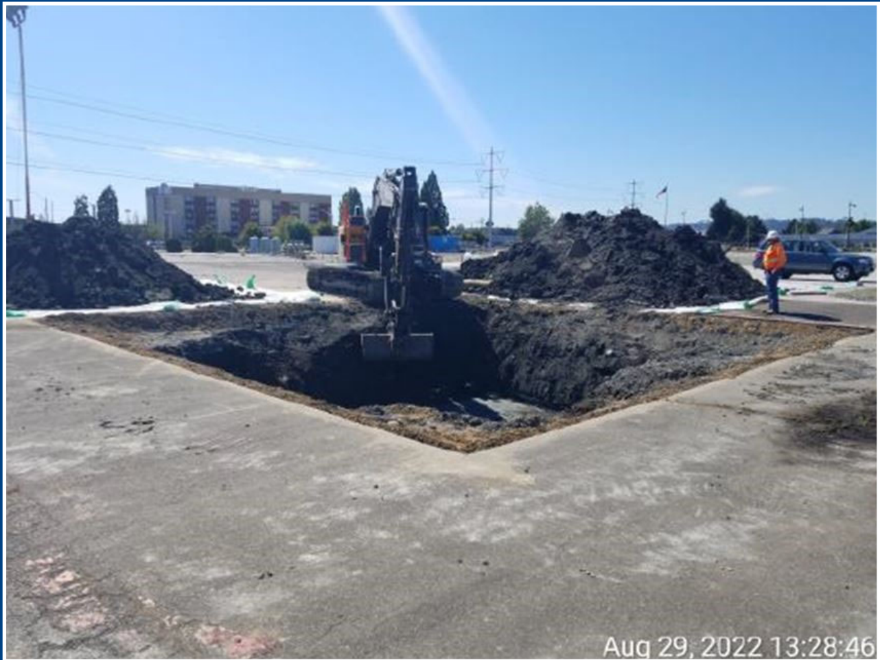
Stride BRT Environmental Remediation Work at South Renton Transit Center
