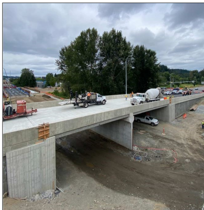
Pave and get ready to open 202/520 on-ramp to through traffic
