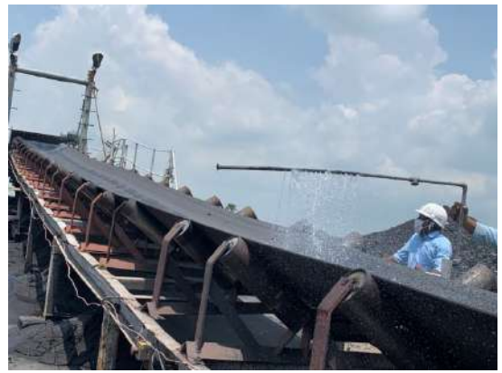
Image: Water sprinklers arranged all along the belt To control the production of dust.
