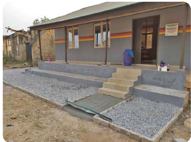
Library upgrade at UMC Primary School, Ibadan
