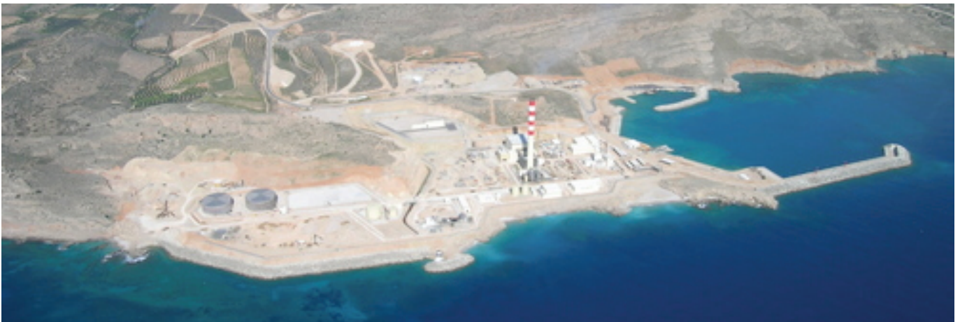
Atherinolakkos Power Plant aerial view
