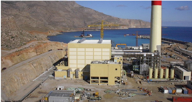
General view of the Atherinolakkos Thermal Power Plant
