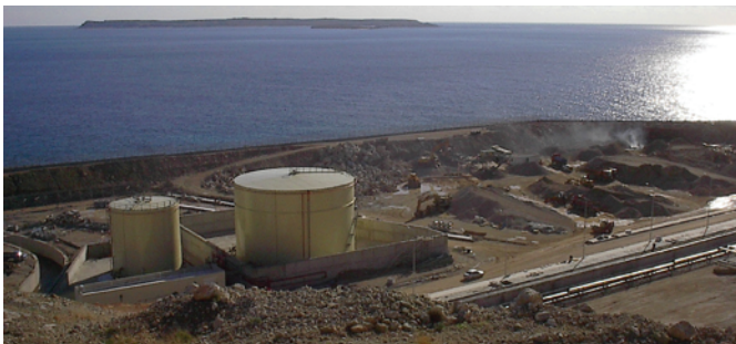
Southern coast of the Power Plant
