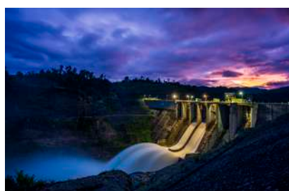
Hydropower Plant Hua Na (Nghe An)
