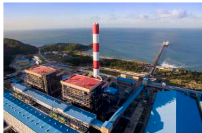
PetroVietnam Vung Ang Power Company (Ha Tinh)
