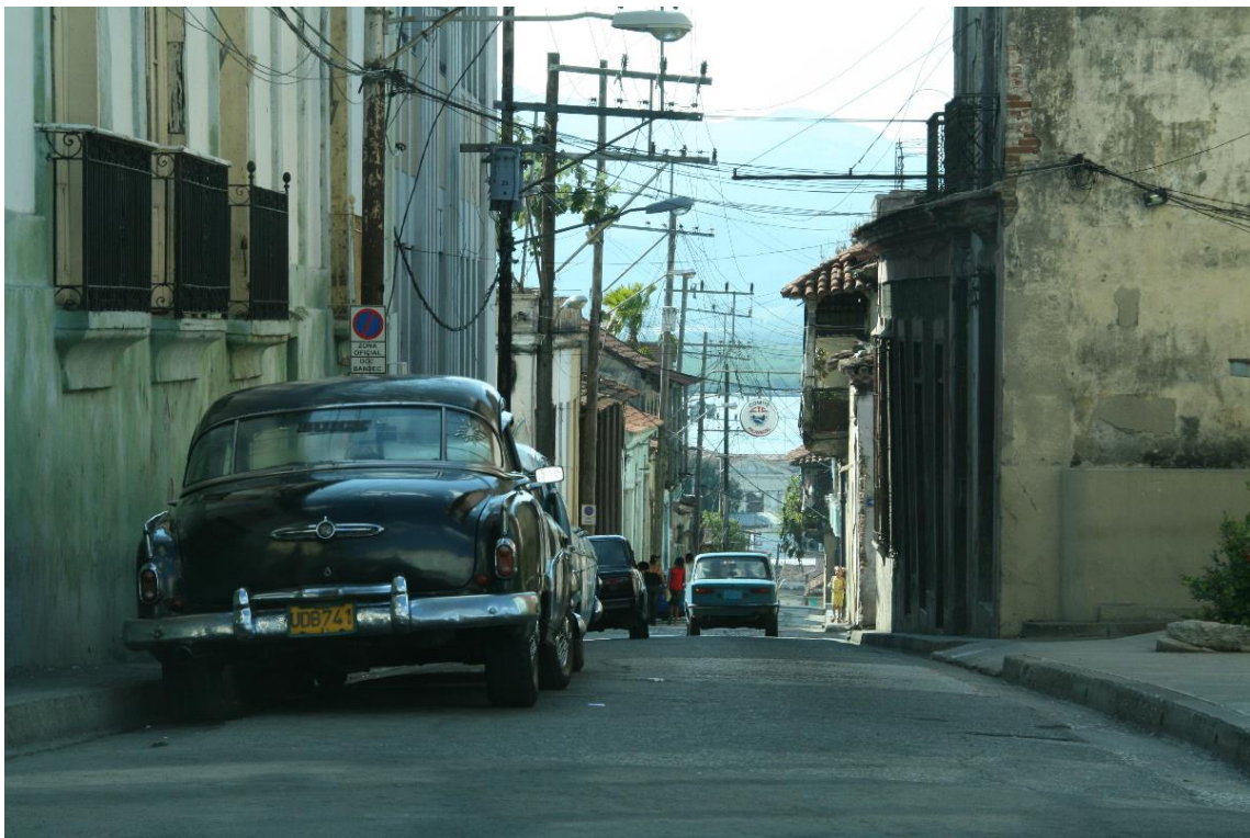
Local electricity grid, Santiago de Cuba
