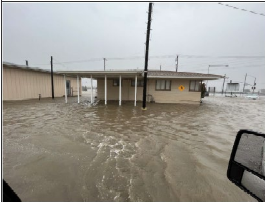
This Photograph Shows: Flooded yard
