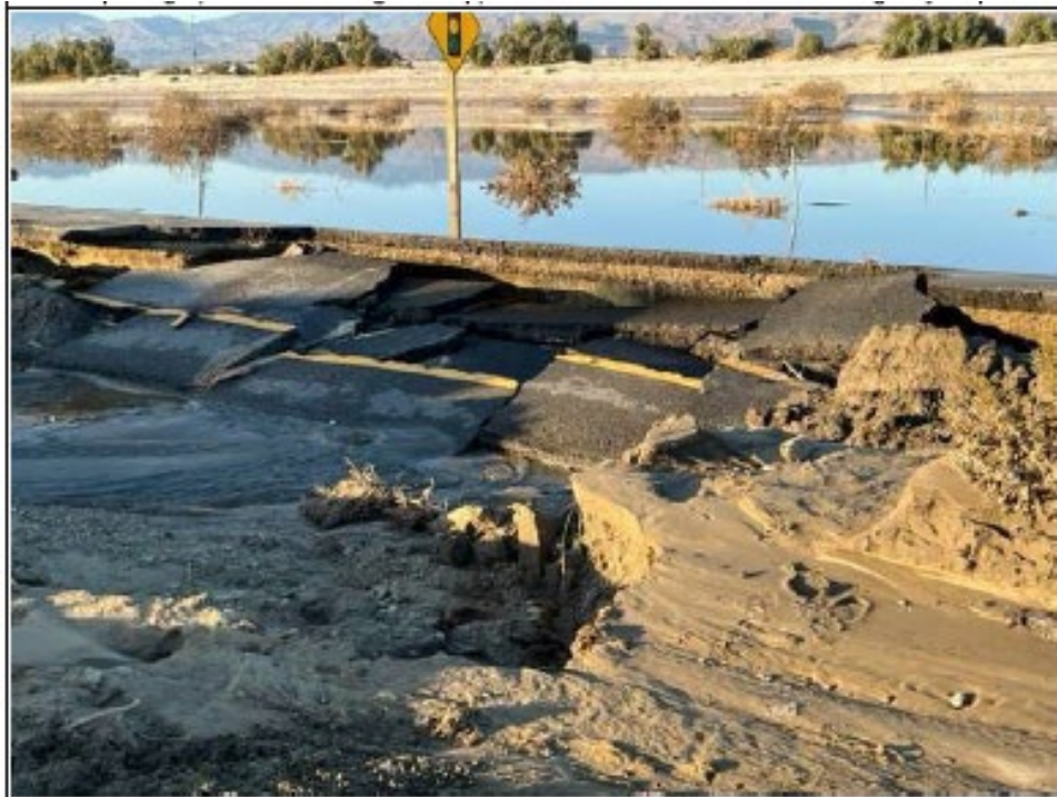
This Photograph Shows: I-10 Eastbound Exit Ramp
