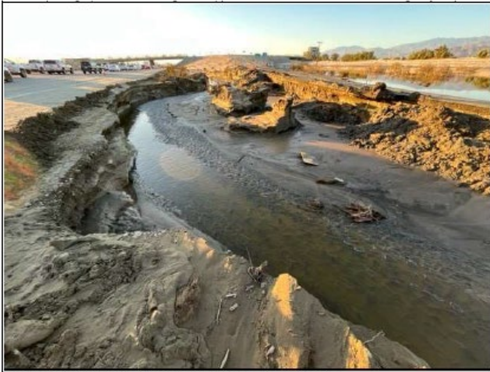
This Photograph Shows: I-10 mainline and Eastbound Exit Ramp
