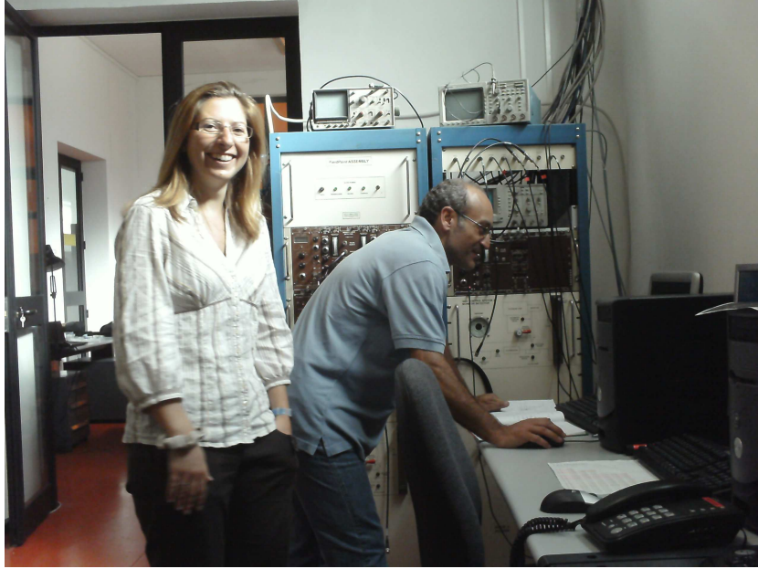
Figure 8.24: Control room of XACT
