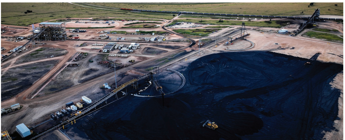
The Run Of Mine stockpile at Carmichael.
