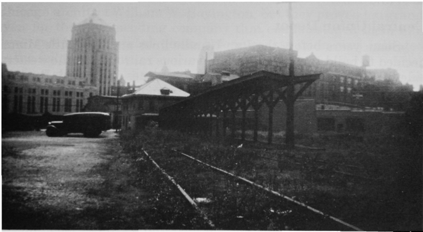
Fig. 21. Court Street Station, platform and canopy. From the private collection of William C. Pletz; reproduced with permission.
