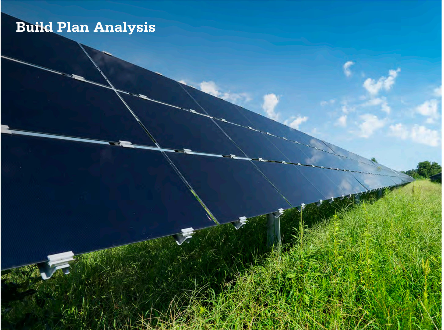
Springfield Solar Facility; Orangeburg, South Carolina
