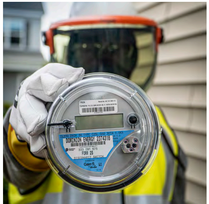
DESC's new smart meter
