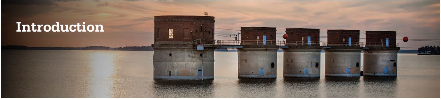
Intake towers at Lake Murray, SC
