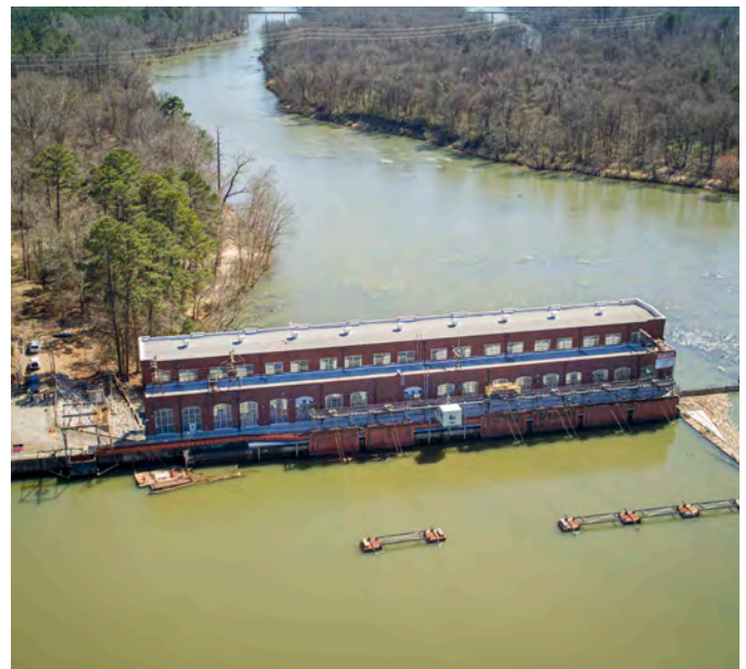
Parr Hydro Station; Fairfield County, SC
