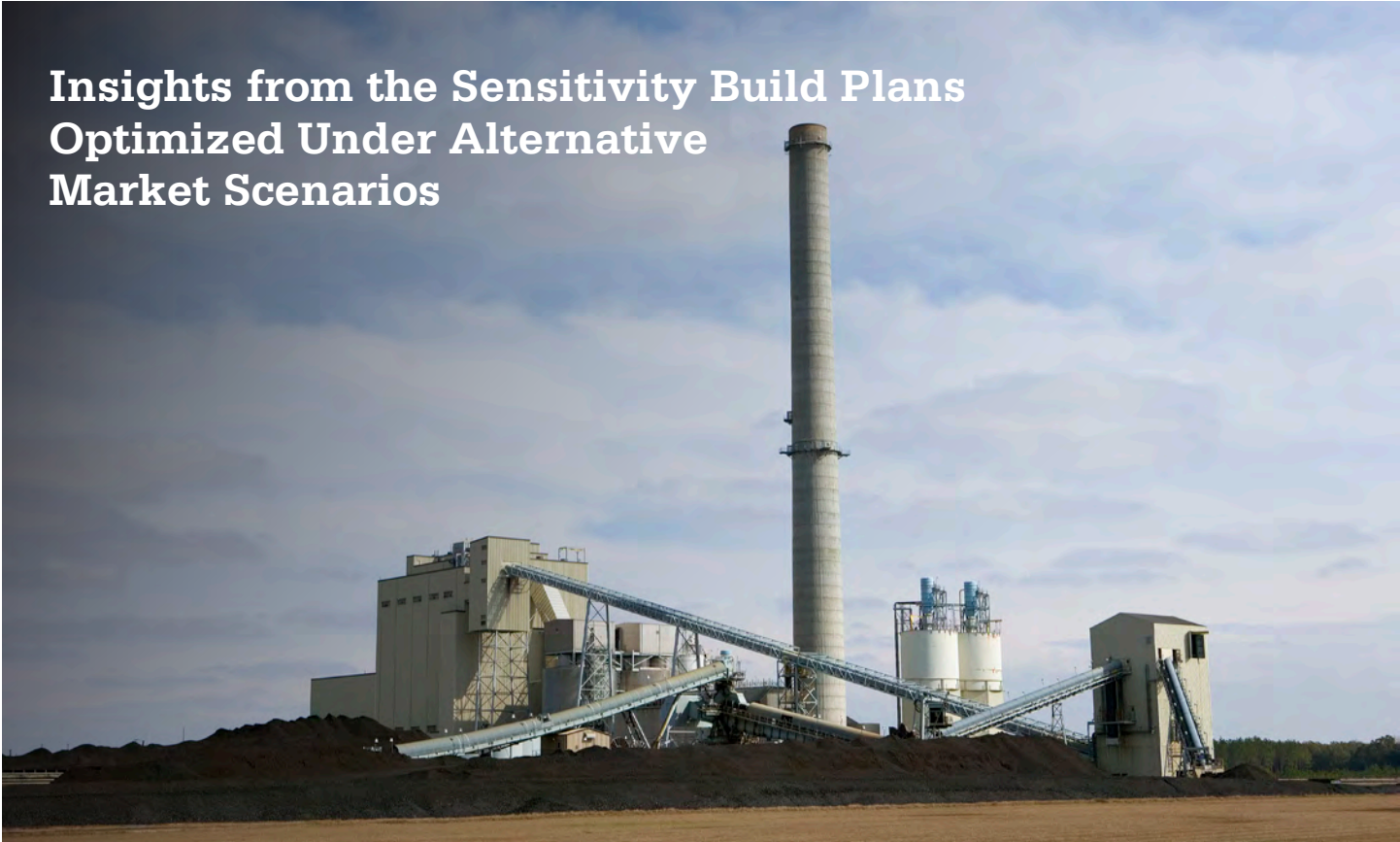
Cope Station; Cope, South Carolina
