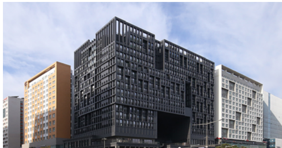
Munjeong-dong Pierre de (Caulking-type panels)
