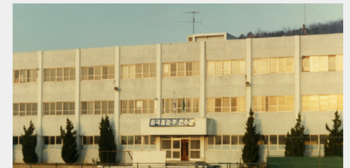
Dongkuk Steel's Group HRD Center in Busan
