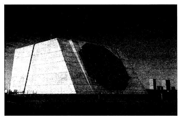
Perimeter Acquisition Radar (PAR) at the Grand Forks site. This radar provided long range warning and acquisition for the Spartan missile. Credit: US Army Space and Strategic Missile Command
