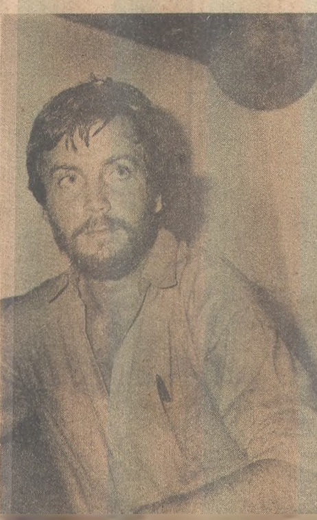
José Luiz coordena as obras
