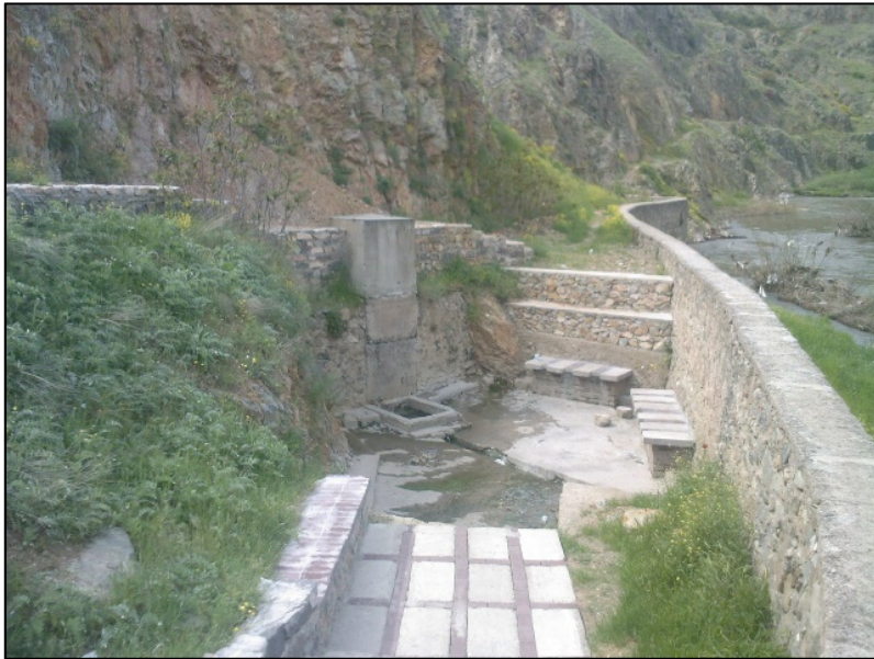
Fig. 9. Geothermal spring Ldži, near Shtip
