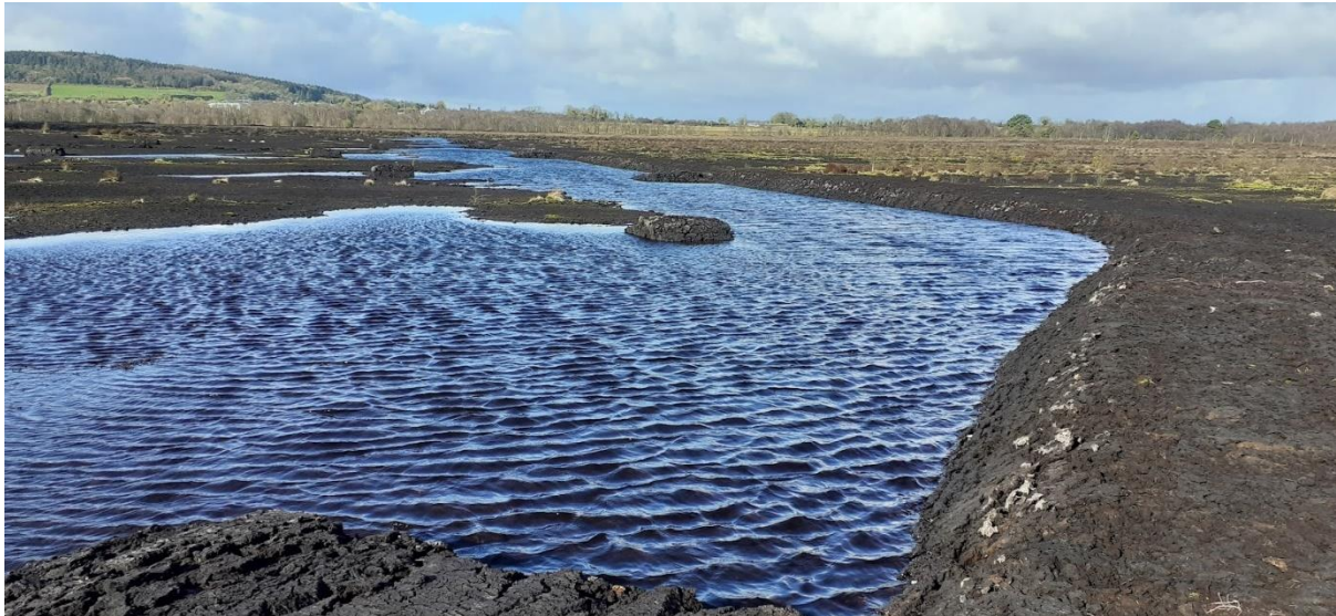
Figure 2.4 Example of existing cell bund constructed at Mouds Bog SAC
