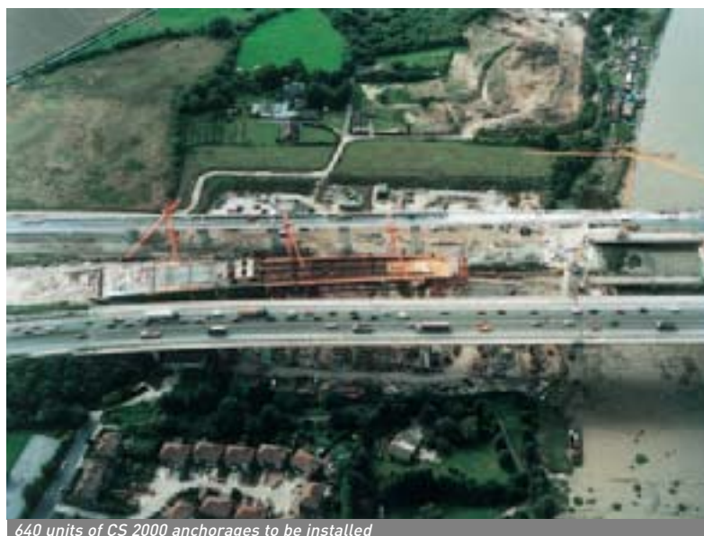
640 units of CS 2000 anchorages to be installed
