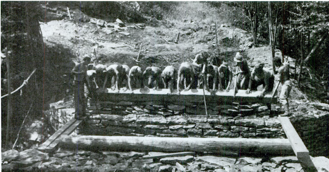
Figure 15--CCC enrollees building a bridge at Mineral Springs, PA, 1935. National Archives 35-6-4343)
