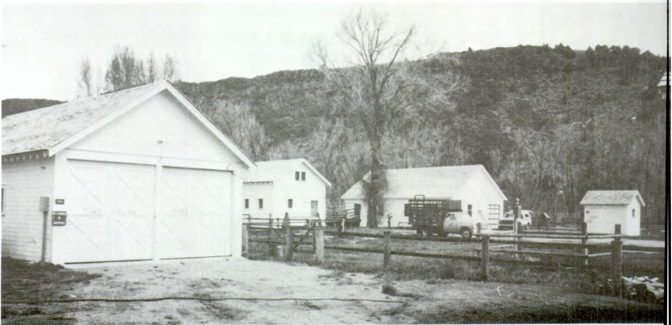
Figure 132--From left to right: Snake River Administrative Site Fire Cache (Building 3), Barn (Building 5), Warehouse (Building 6), and Gas House (Building 8).
