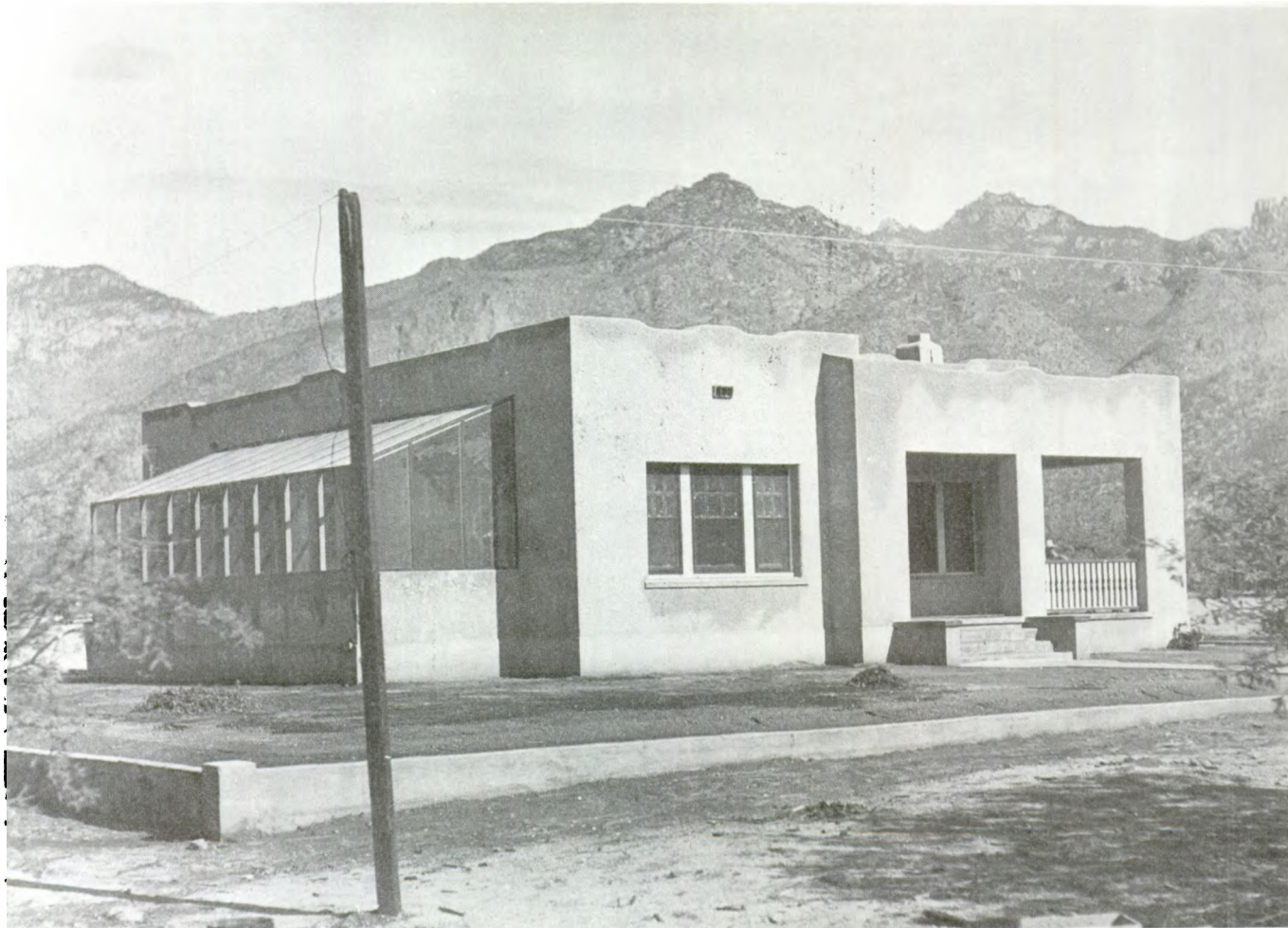
Figure 126--Dwelling, Lowell Ranger Station, Coronado National Forest, AZ. (National Archives 95-G-292457)
