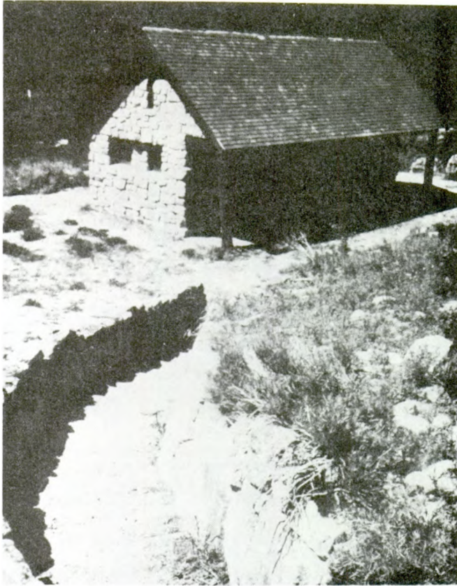
Figure 12--Bathhouse, Sunbeam Hotsprings, Sawtooth National Forest, ID.
