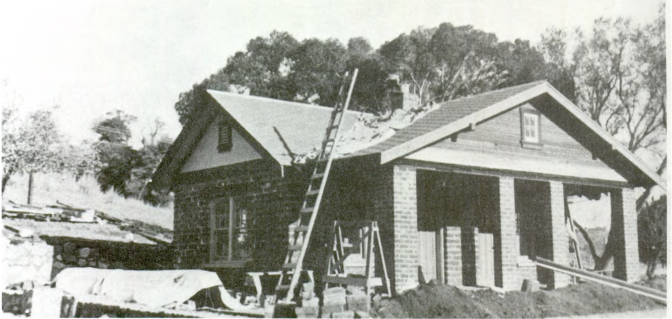
Figure 116--Office, Canelo Ranger Station, under construction in 1933, Coronado National Forest, AZ.
