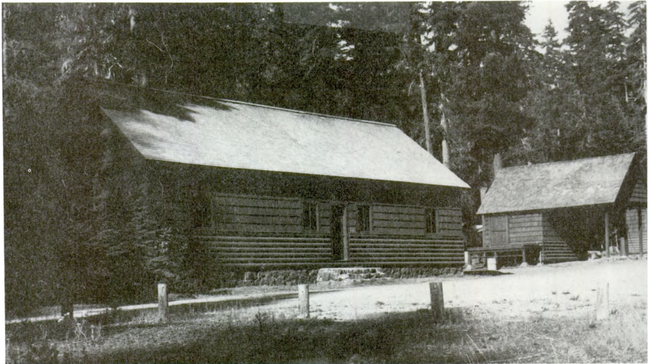
Figure 95--Fire warehouse, Clackamas Lake Ranger Station, Mount Hood National Forest, OR. (Photo by William D. Honey, 1982)
