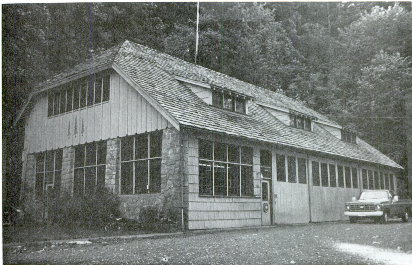
Figure 104--Warehouse, Columbia Gorge Ranger Station, Mount Hood National Forest, OR. (Photo by Dennis Egner, 1982)
