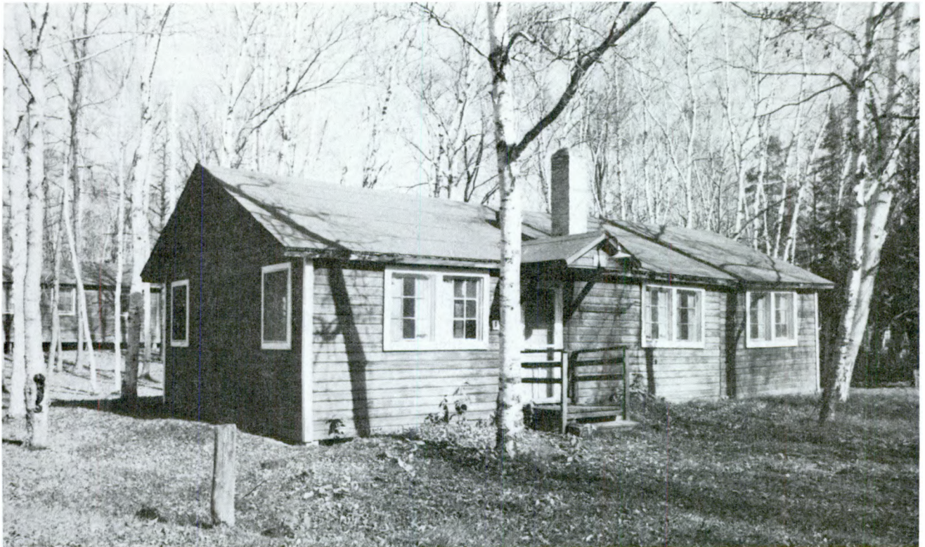
Figure 26--Another view of Rabideau CCC camp, Blackduck Ranger District, Chippewa National Forest, MN.
