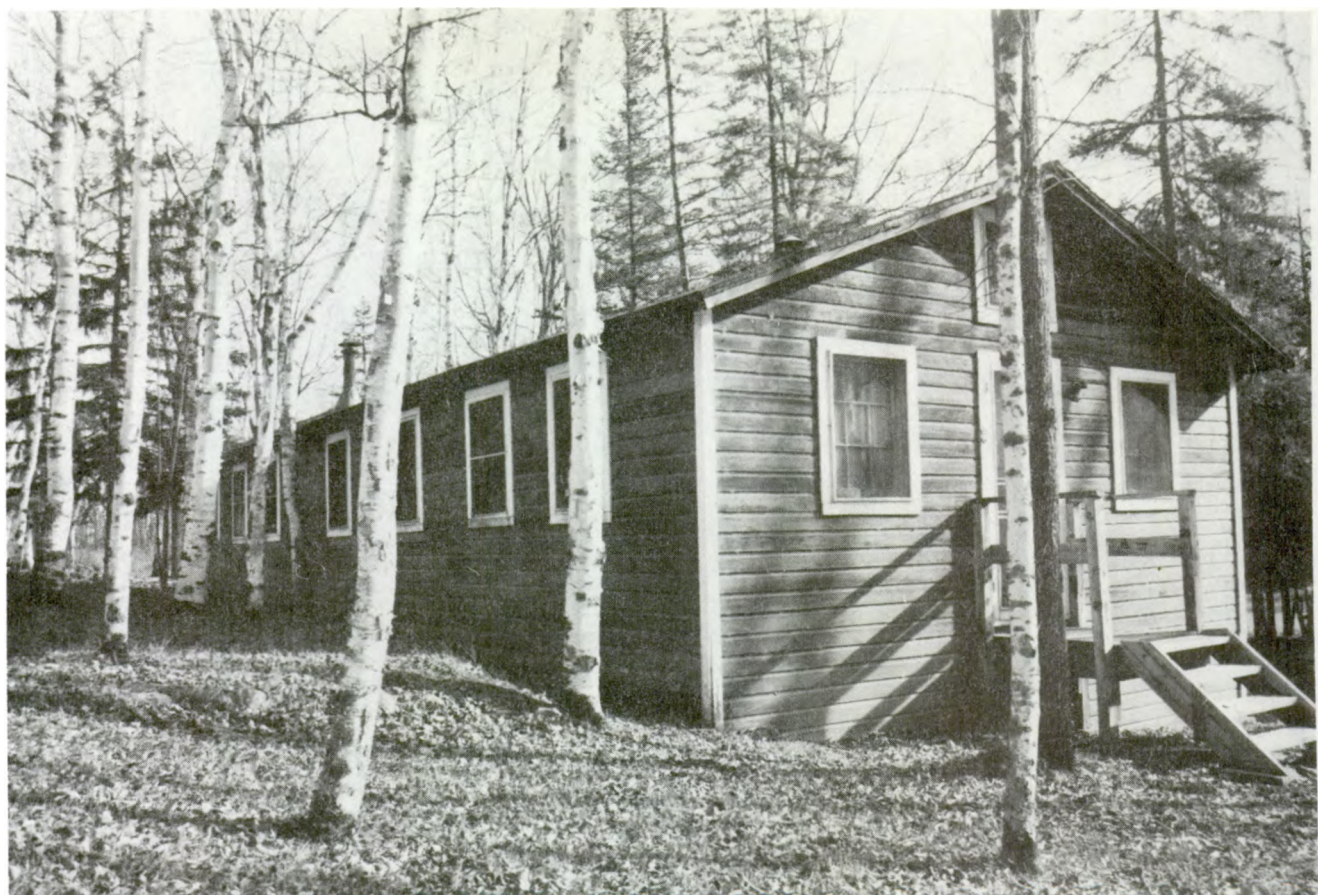
Figure 25--Rabideau CCC camp, Blackduck Ranger District, Chippewa National Forest, MN.
