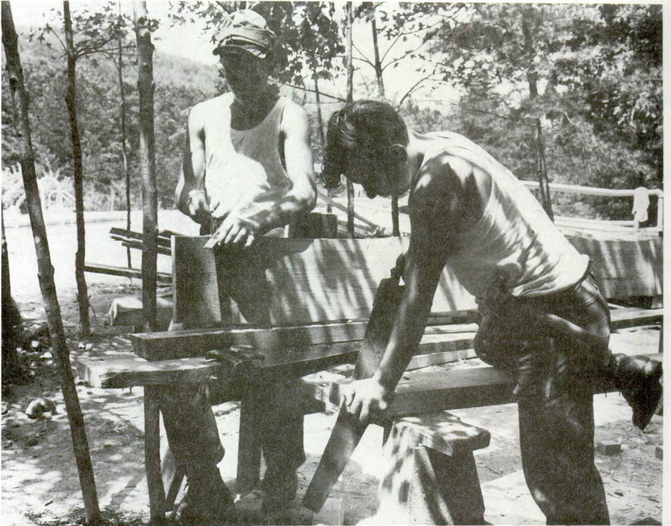
Figure 50--Camp Roosevelt CCC enrollees making waney-edge siding for Powell's Fort campground. (National Archives 35-G-625)
