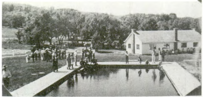
Figure 7--Bessey swimming pool, Nebraska National Forest.
