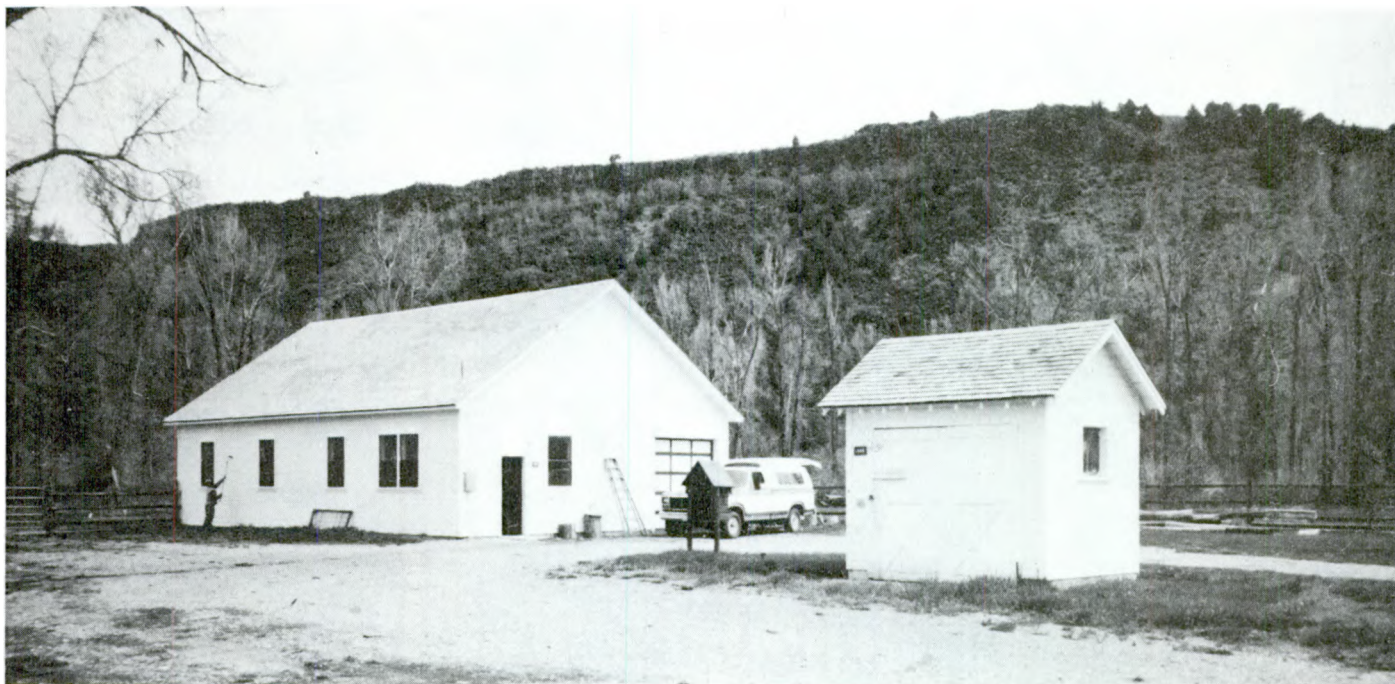
Figure 136--Snake River Administrative Site Warehouse (Building 6, at left) and Gas House (Building 8).
