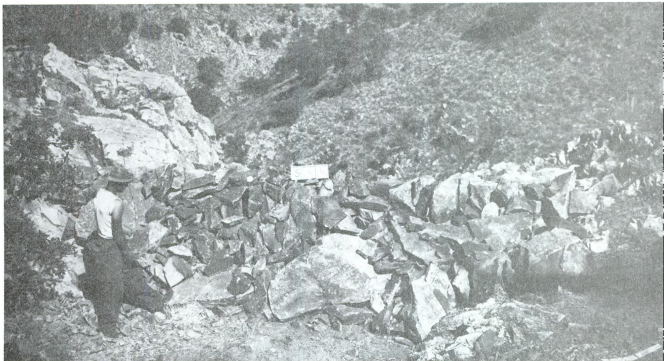
Figure 119--Stream control dam constructed by CCC Camp F-30 during winter 1933-34 on Santa Rita Experimental Range, AZ. (National Archives 95-G-298650)
