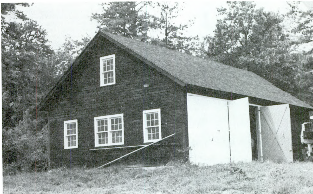
Figure 58--Garage at Sherando Lake, built in 1933-34, that was formerly part of Sherando CCC camp and is now used as Forest Service equipment shed. (Photo by Alison T. Otis, 1982)
