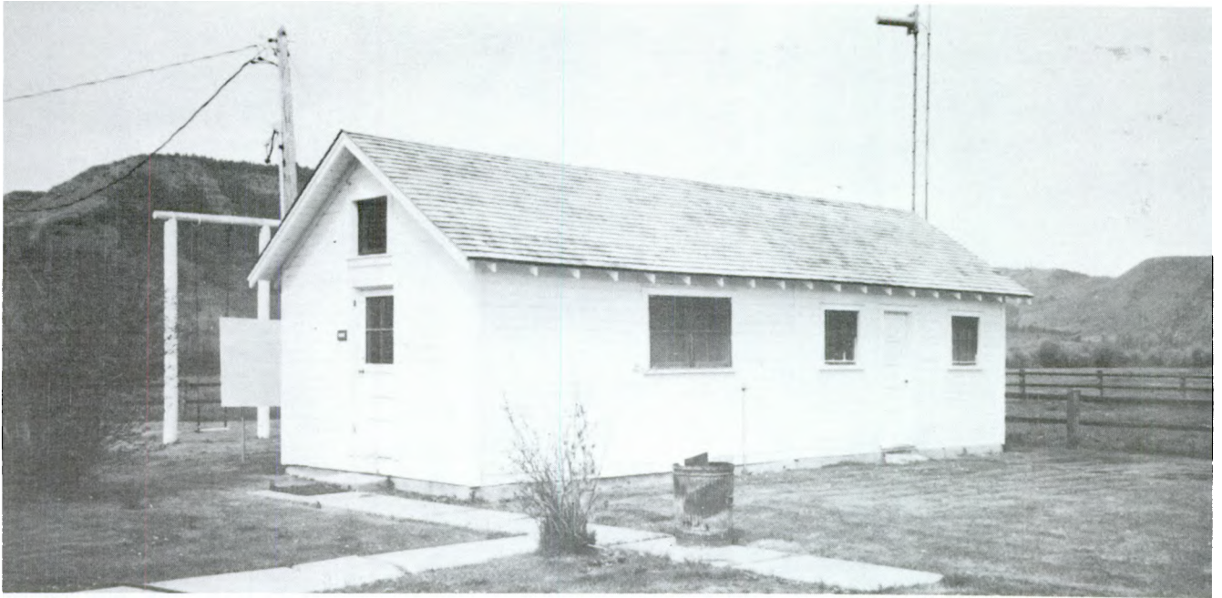
Figure 133--Snake River Administrative Site Office (Building 4). The original woodshed forms the left half of the existing structure.
