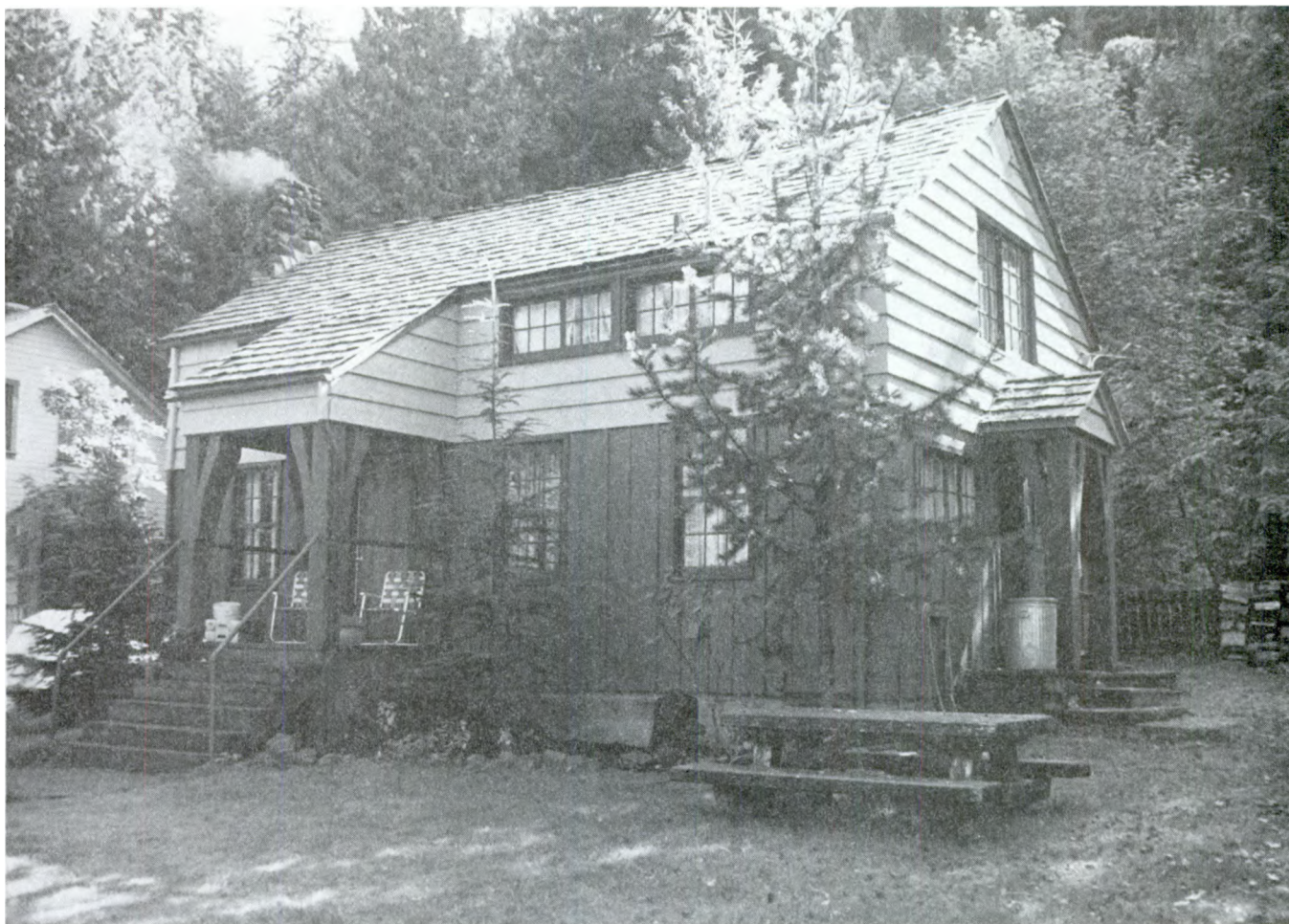
Figure 86--Bunkhouse/residence, Zigzag Ranger Station, Mount Hood National Forest, OR. (Photo by Dennis Egner, 1982)
