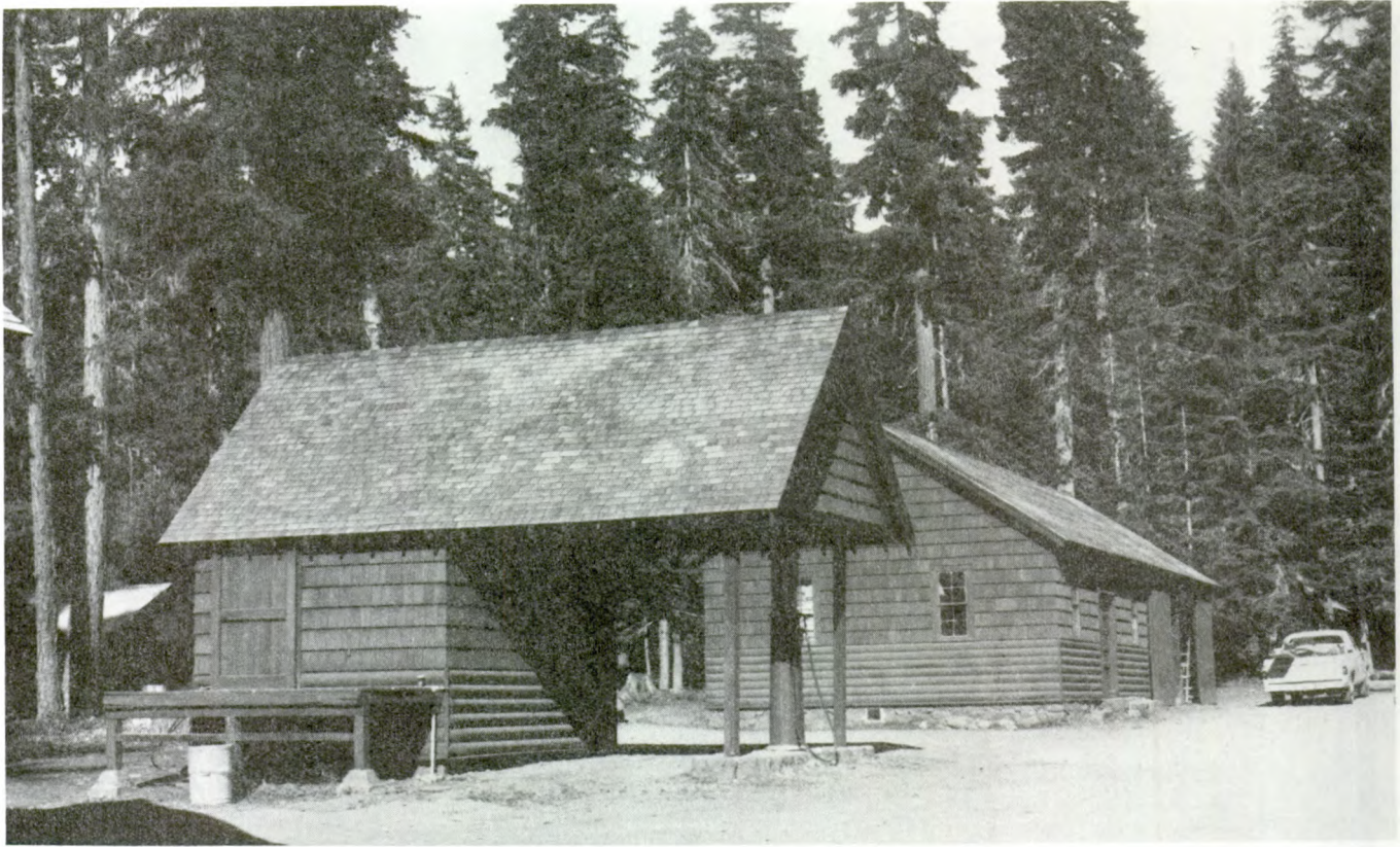
Figure 97--Gas and oil house with roads and trails warehouse in background, Clackamas Lake Ranger Station, Mount Hood National Forest, OR. (Photo by William D. Honey, 1982)
