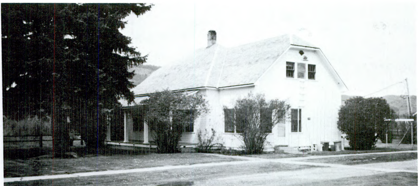
Figure 130--Snake River Administrative Site Dwelling (Building 1), looking west.
