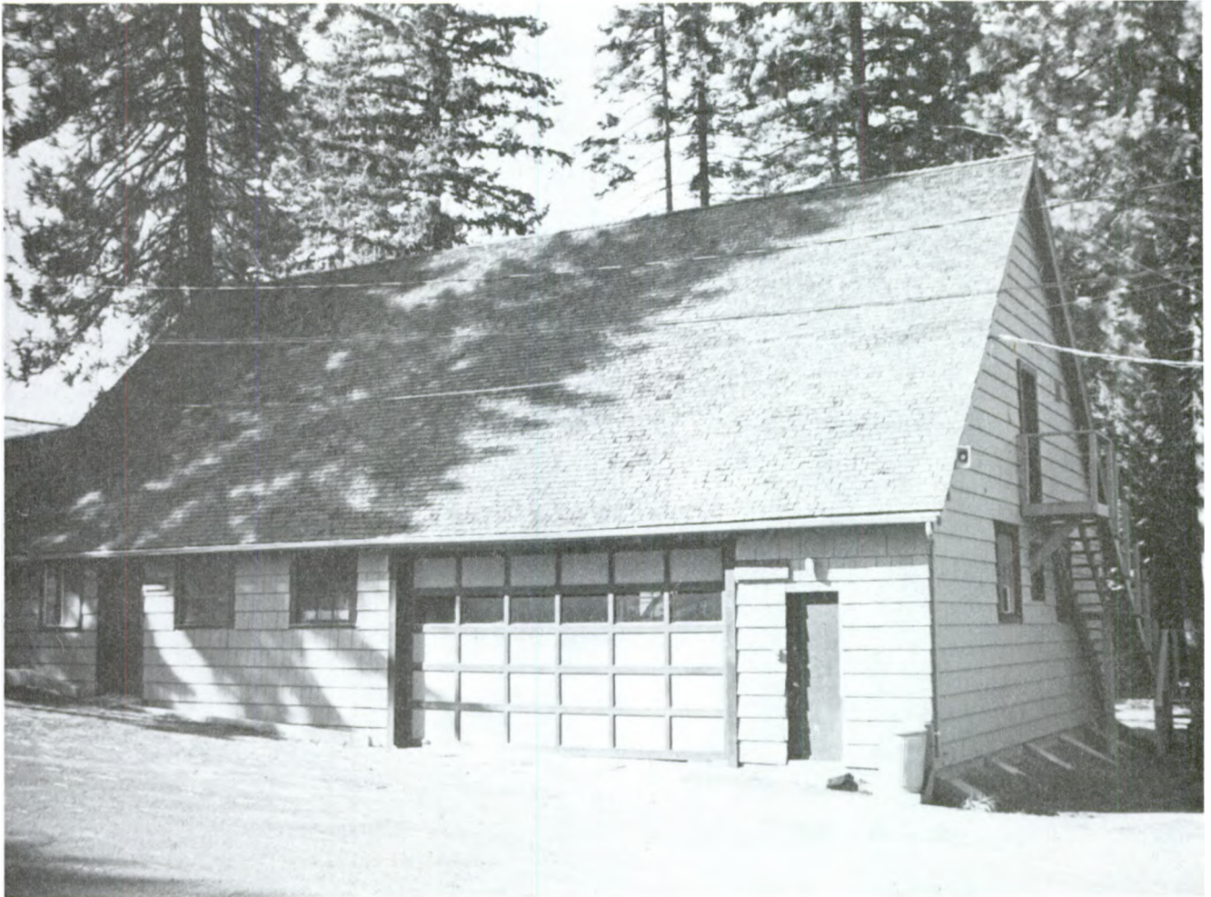
Figure 82—Machine shop/storage building, Parkdale Ranger Station, Mount Hood National Forest, OR. (Photo by Dennis Egner, 1982)
