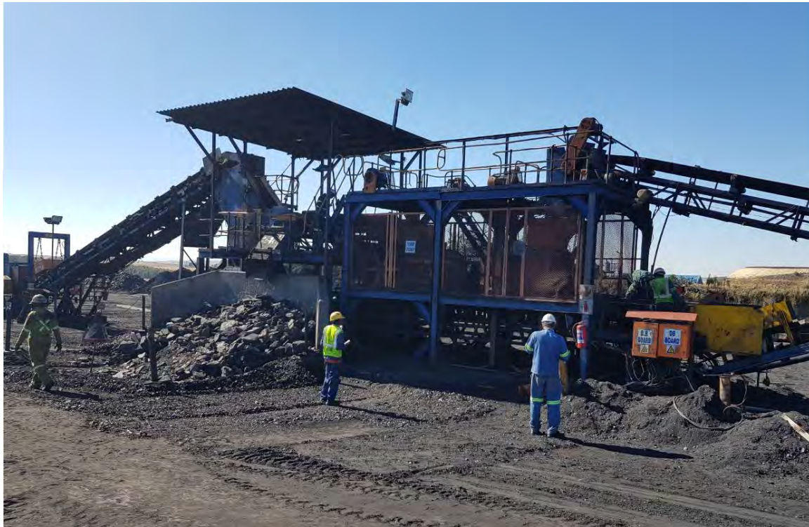
FIGURE 3-3: EXAMPLE OF A TYPICAL WASH PLANT
