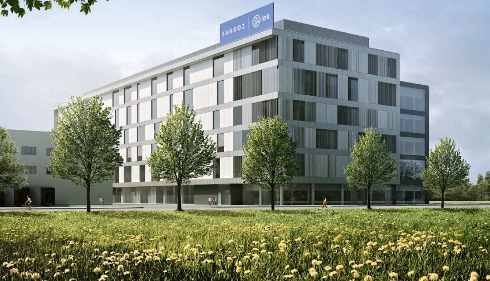
Architect's render of our new biologics manufacturing plant in Lendava, Slovenia, expected to be operational in 2026.
