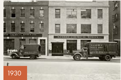
1930 Warehouse, New York
