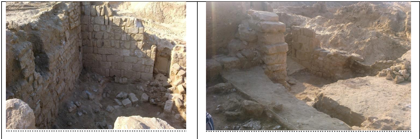
Damage to the old port of Gaza - Al-Balahiya, Gaza.
